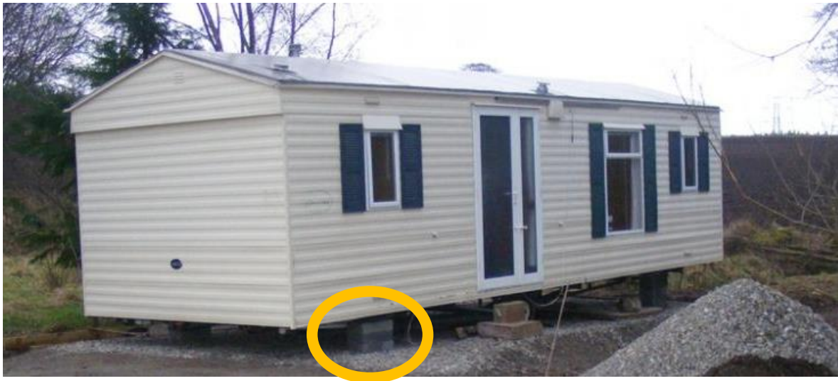
Figure 4, example of the removable concrete blocks to be used to level the temporary caravan
