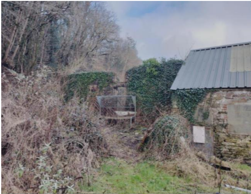
Figure 2, Photo showing south elevation of the old farmhouse
