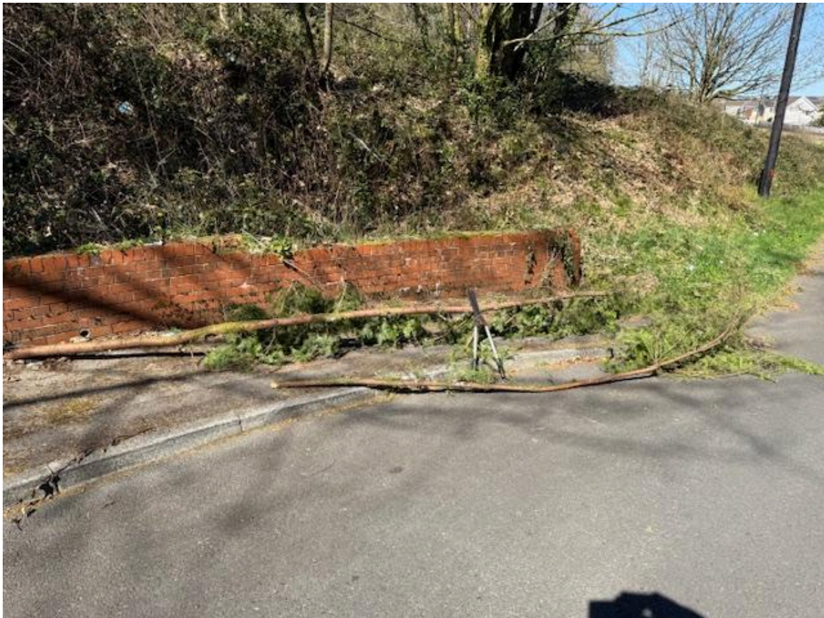
IMAGE A: Some of the fractured branches
