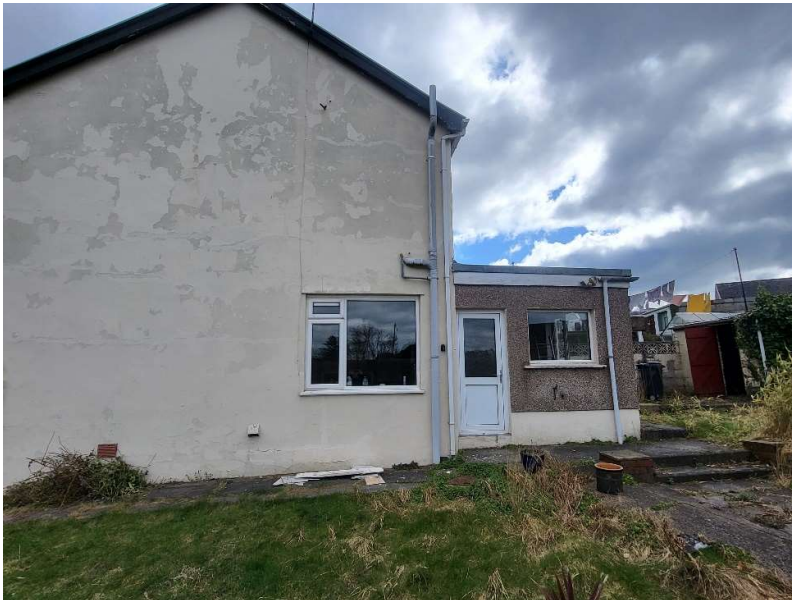
Side elevation view of property where new extension will be positioned above existing ground floor area. Lawned areas can be seen.
