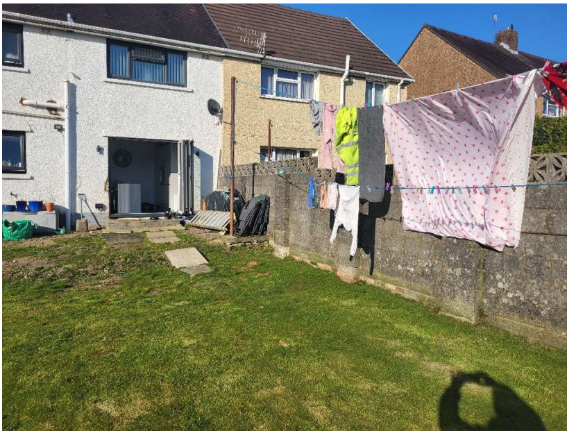
View of rear of existing property showing blockwork boundary wall and rear lawned area.
