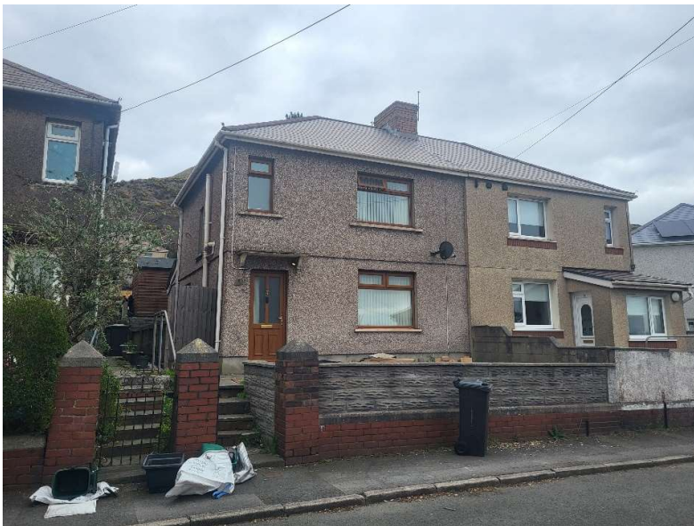
Front elevation view with front access steps to small, raised yard area
