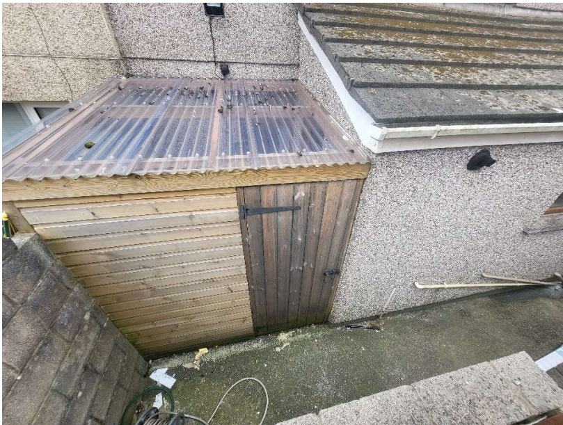
Area where the extension will be built is currently an enclosed timber stores/utility space
