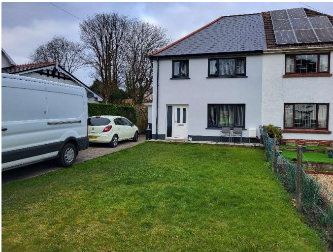
Front elevation, which will remain unchanged. Post and wire boundary to attached neighbour and be seen with large lawn and concrete driveway
