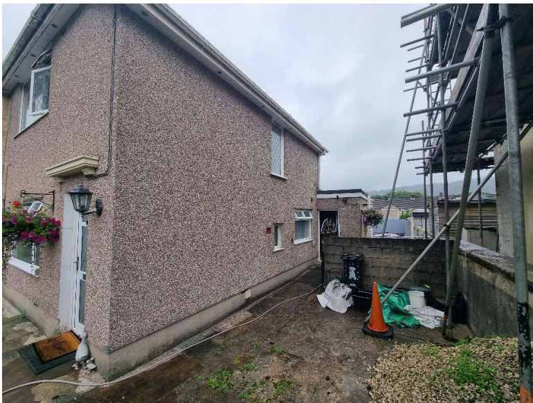
View of side elevation where there is an existing side extension. This is area where the new extension will be sited. Stonework boundary wall in place.
