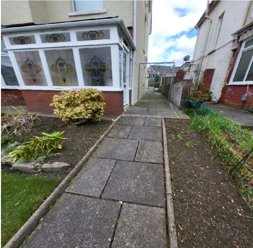
View down the side elevation of the property including a concrete paved path and brickwork boundary wall to neighbour. Bedding areas shown and these will remain.
