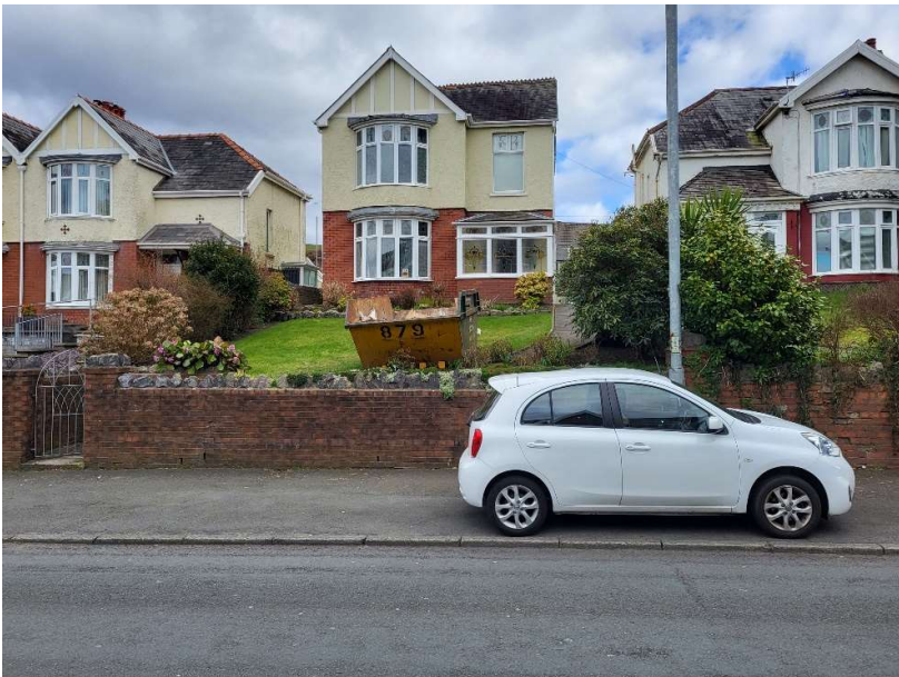
Front elevation of property including existing brickwork boundary wall to highway, large lawn and concrete steps and path to front door.
