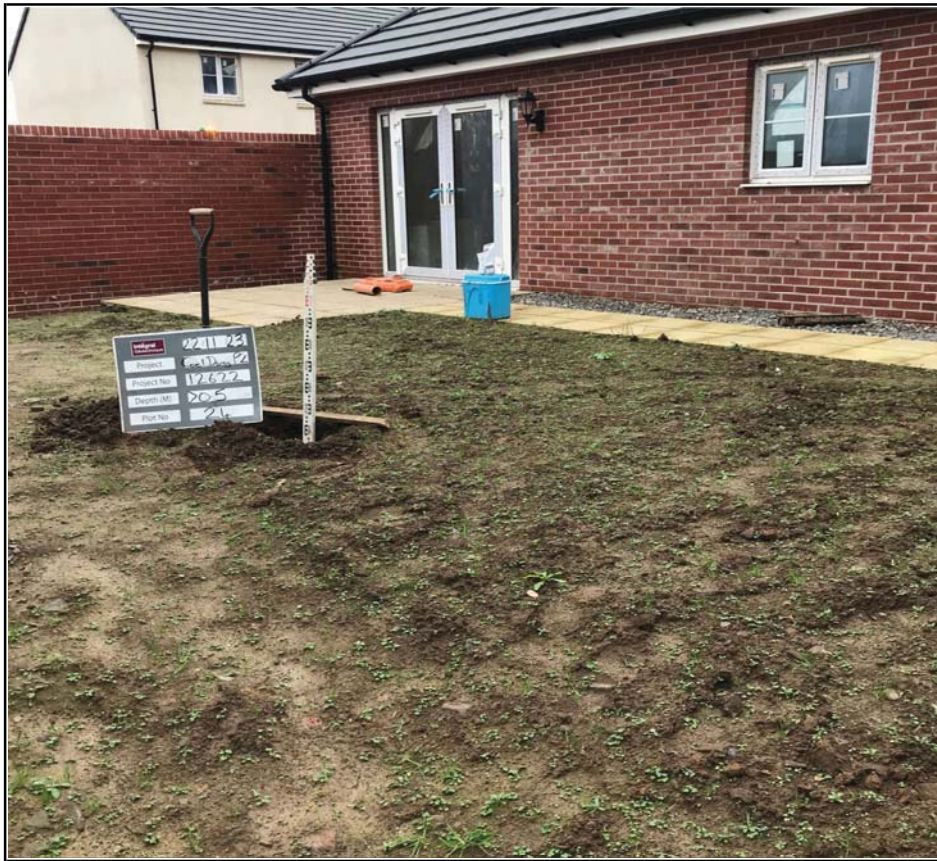
Plot 24 Capping Validation Depth Check
