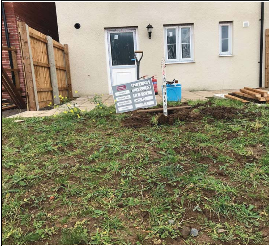
Plot 12 Capping Validation Depth Check
