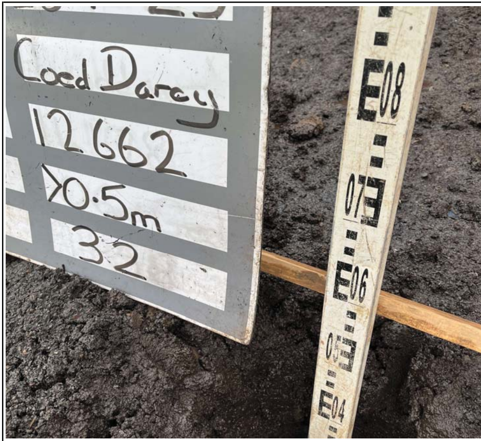
Plot 32 Trial Pit Depth Verification
