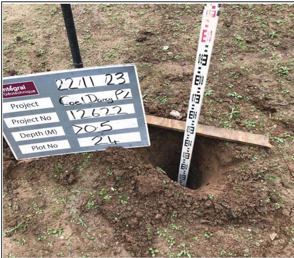
Plot 24 Excavation Trial Pit
