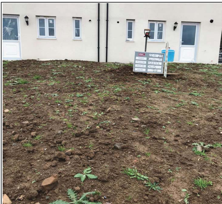
Plot 28 Capping Validation Depth Check
