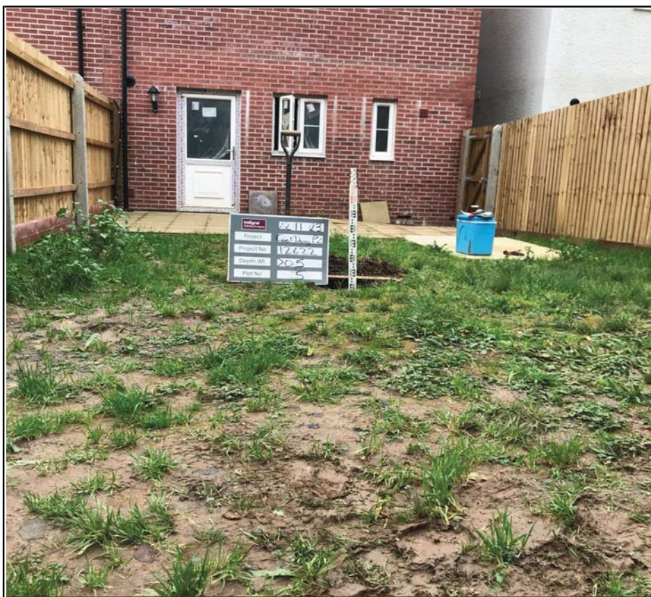
Plot 5 Capping Validation Depth Check
