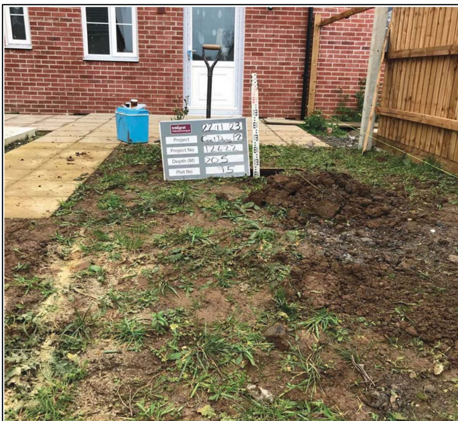
Plot 15 Capping Validation Depth Check
