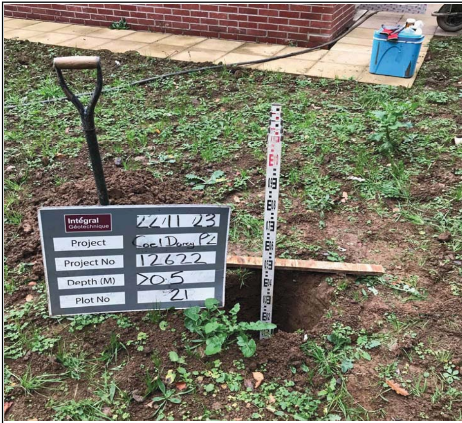
Plot 21 Capping Validation Depth Check
