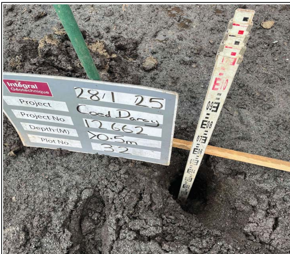
Plot 32 Trial Pit Excavation
