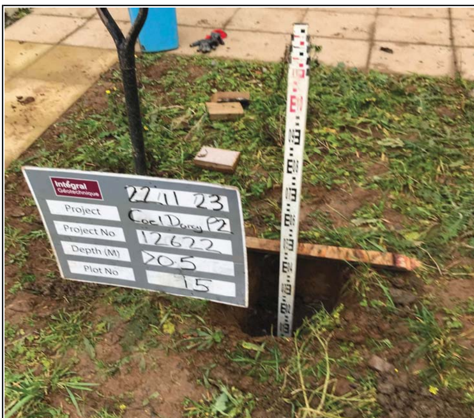
Plot 15 Excavation Trial Pit
