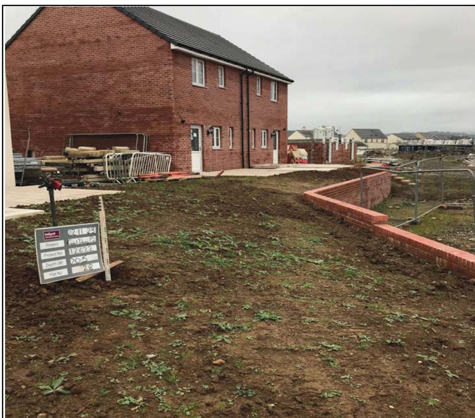
Plot 28 Excavation Trial Pit
