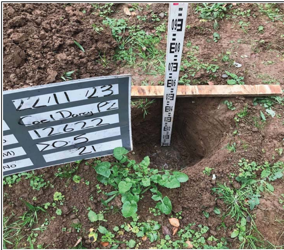
Plot 21 Excavation Trial Pit
