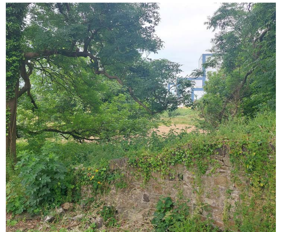
Existing stone wall to western boundary
