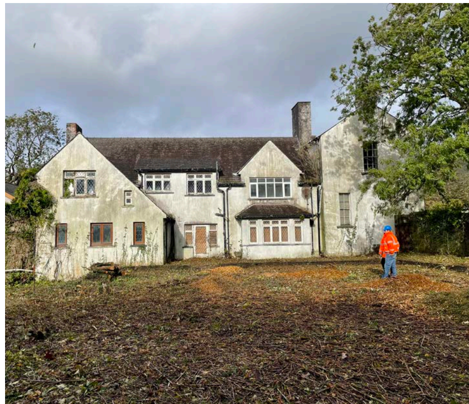
View 06 - View of the southern facade of Tyn-y-Caeau.
