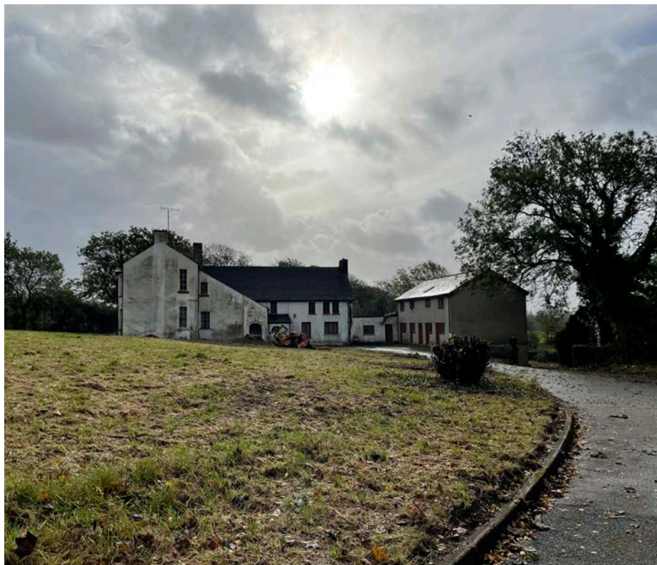
View 05 - View from the centre of the site, towards Tyn-y-Caeau building, located on the southwest part of the site
