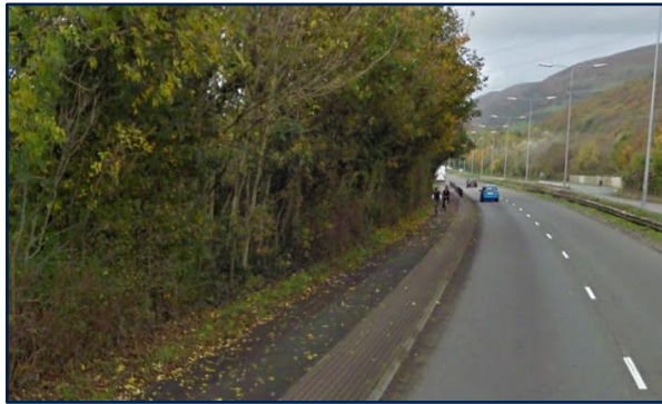
2009 A48 Margam Road Signage
