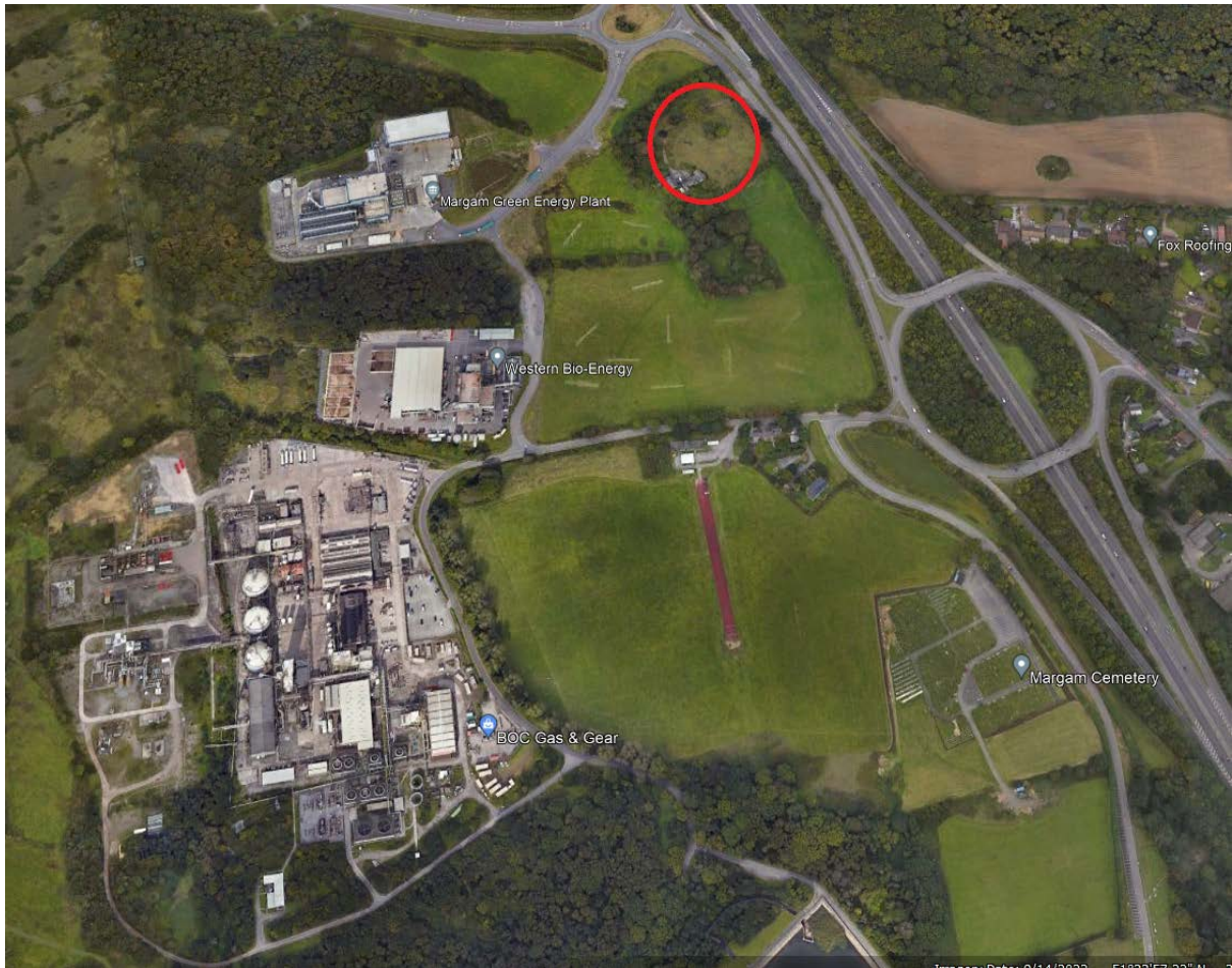
Figure 2. The Site (ringed) relative to the A48/M4 corridor and the three industrial complexes to its west (Margam Green Energy Plant) and south-west (Western Bio-Energy, and BOC Gas and Energy) (Google Earth 2024).
