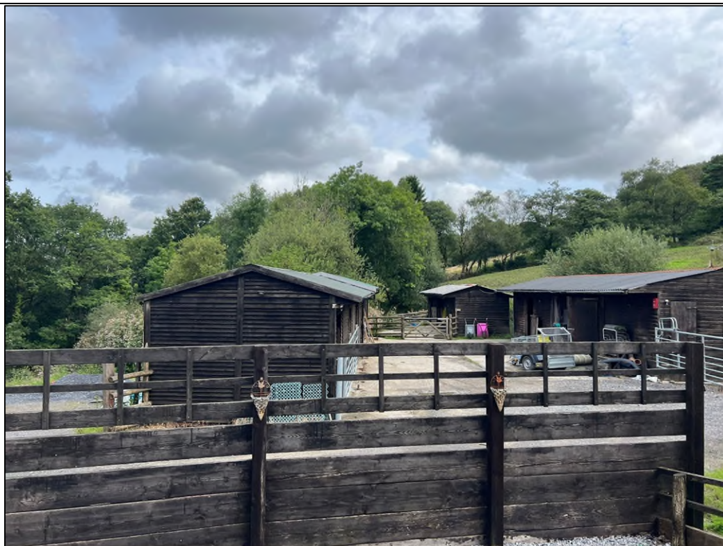
Plate 15 - Stables area at the rear of the house.
