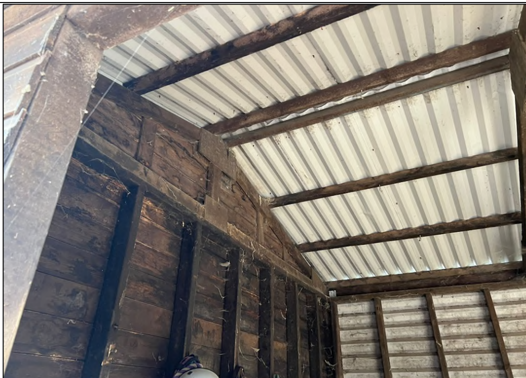
Plate 13 - Inside of the stables with previous evidence of nesting birds.
