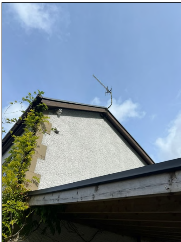
Plate 5 - Southern gable end of the property.
