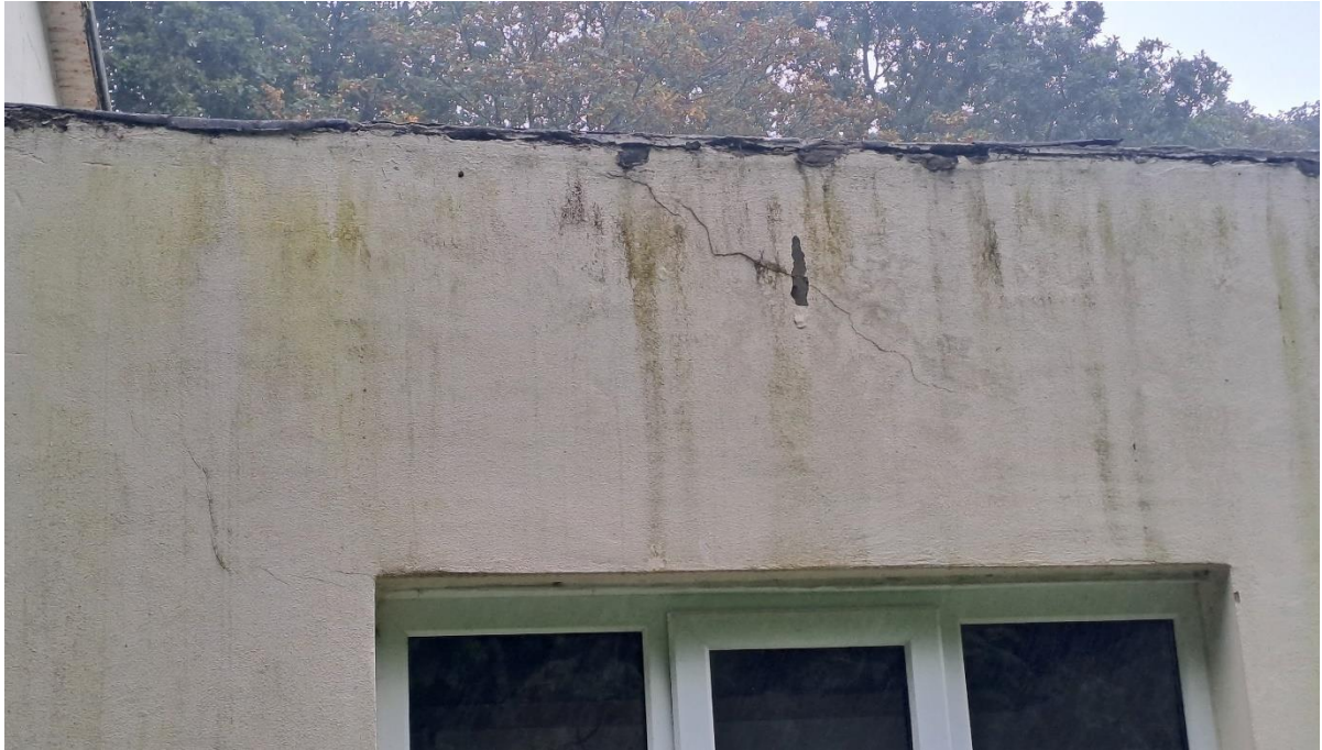
Photograph 9 – Diagonal Cracking
