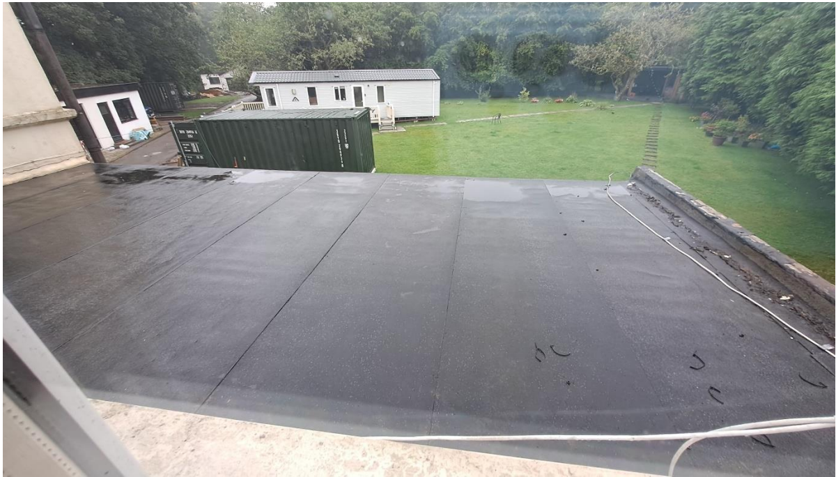
Photograph 21 – Rear flat roof
