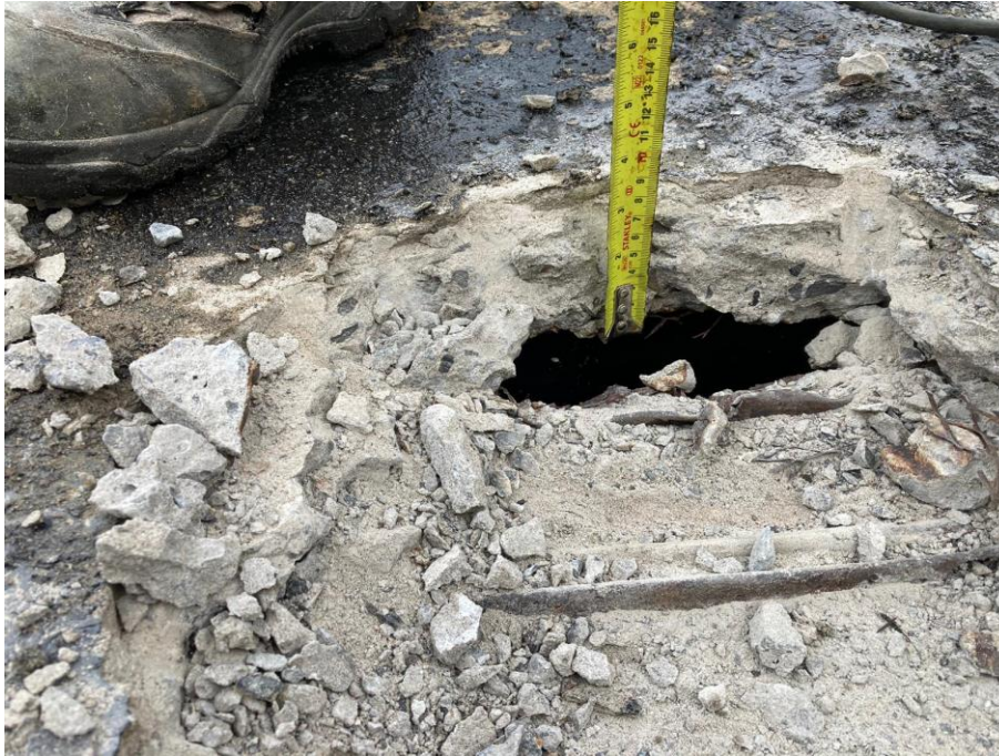
Photograph 23 – Concrete roof depth 80-100mm
