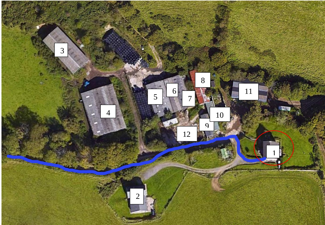
Figure 3 – Pant Howell Ddu Farm building complex
