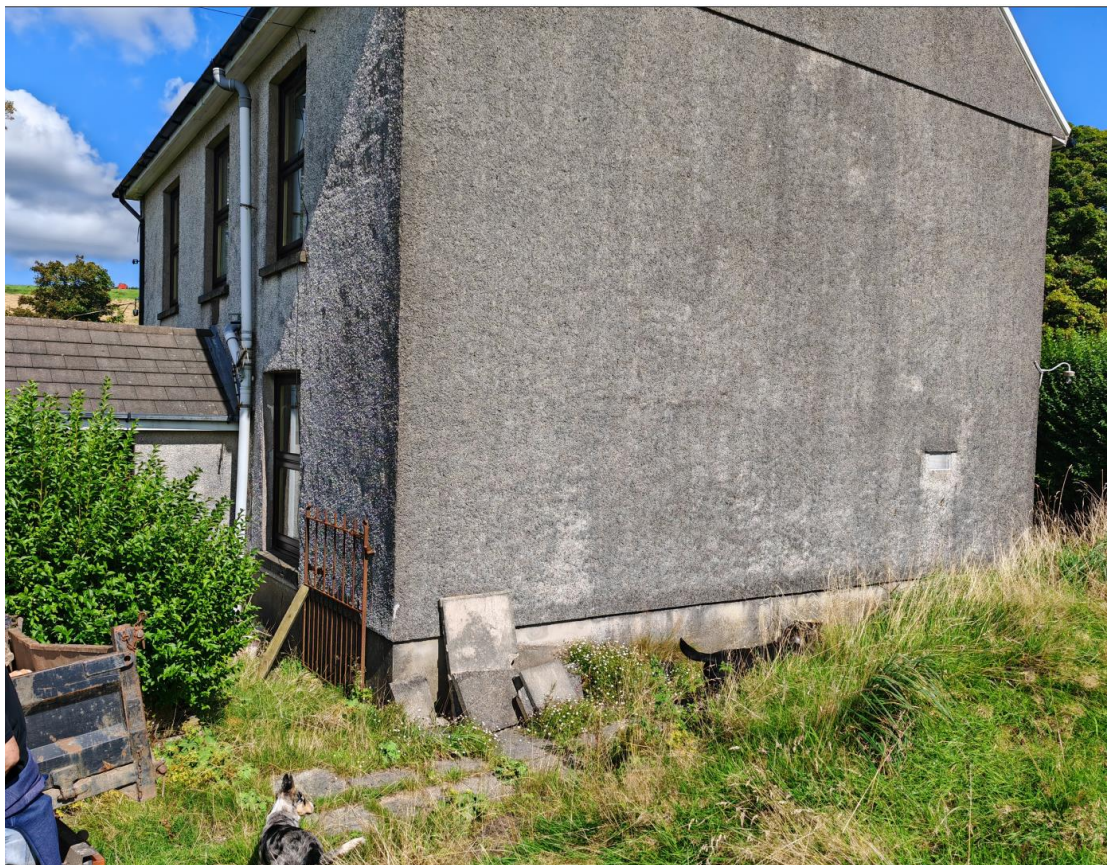
Photo 18 – gable end elevation (south)
