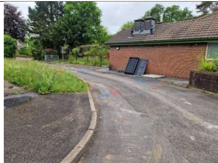
PLATE 02 – Site Entrance – Looking South.
