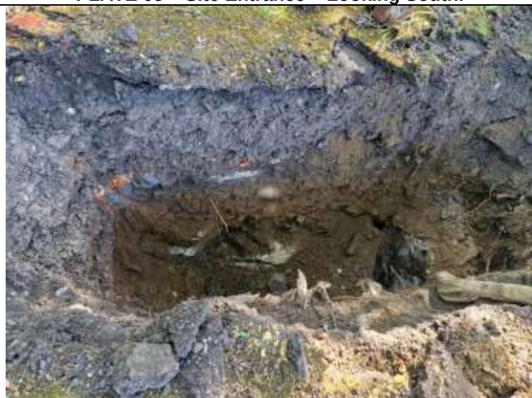
PLATE 07 – Trial Pit Excavation – TP01.
