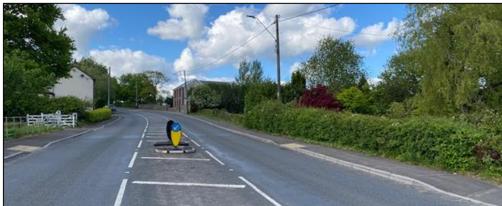
Photo 2 – extent of A road carriageway with site frontage shown lying adjoining continuous lines of adjacent hedgerows
