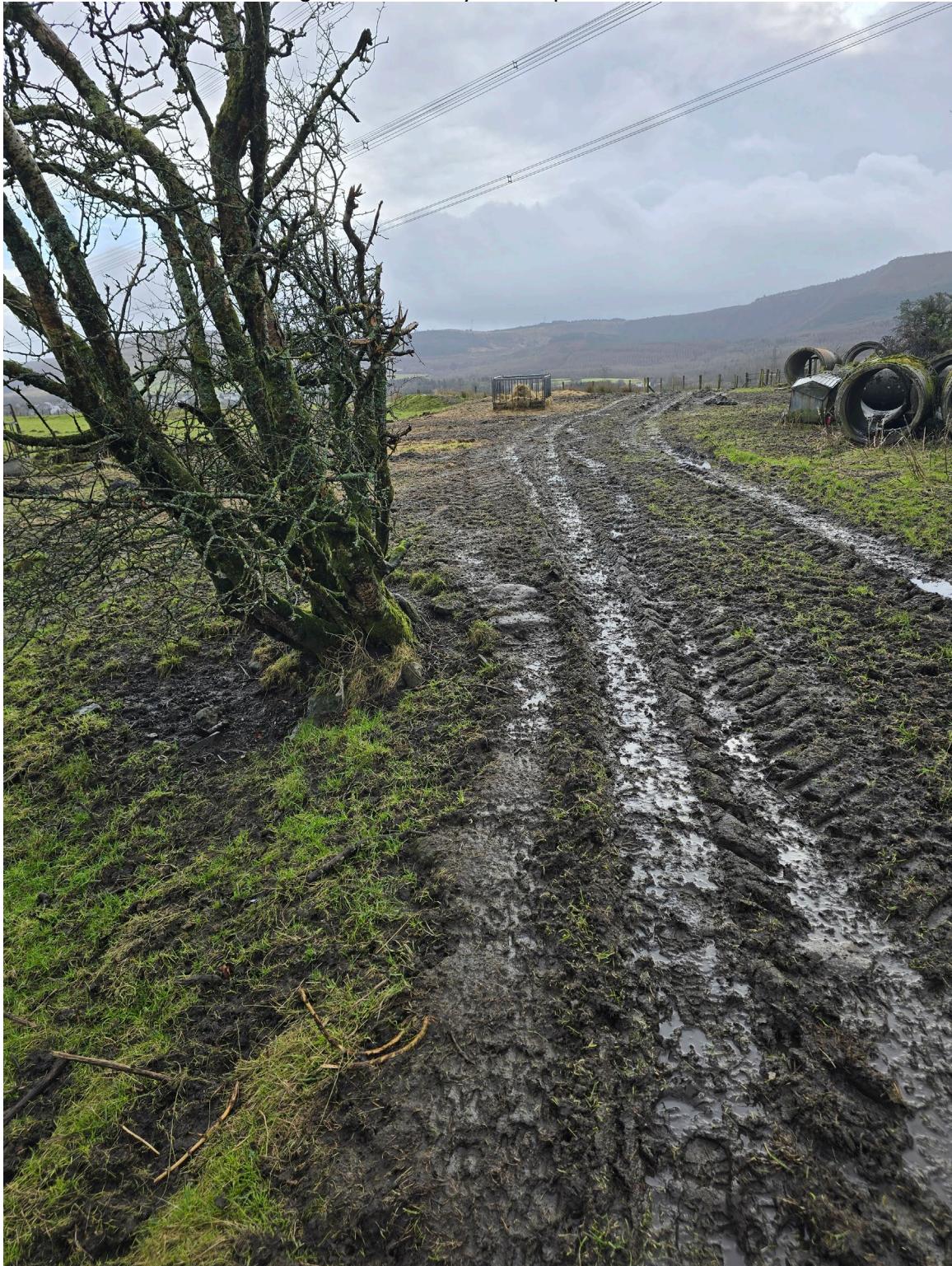
Photo 3: T9 rooting area restricted by the compacted access road to the west.
