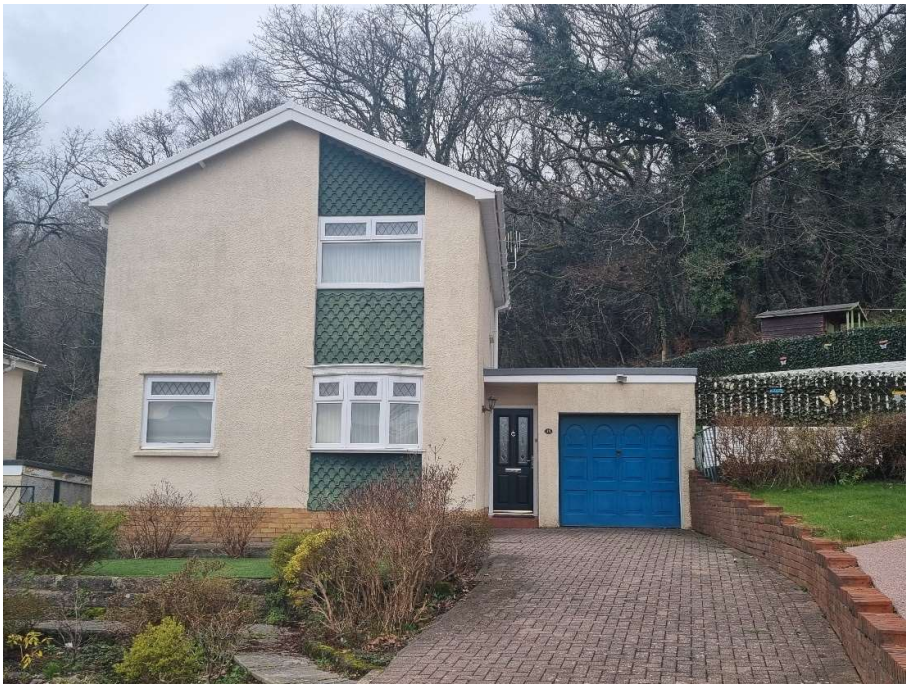
Front elevation view showing brickwork driveway, wall to right hand side neighbours and tiered rockery area
