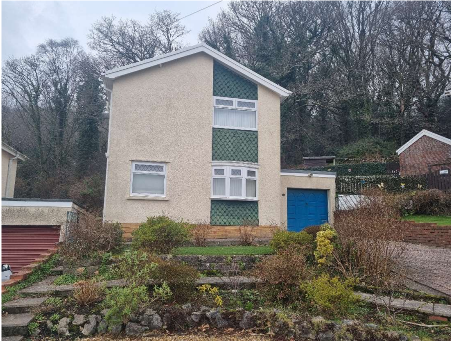
Front elevation view showing tiered rockery area including small lawn and bedding areas with mature shrubbery.
