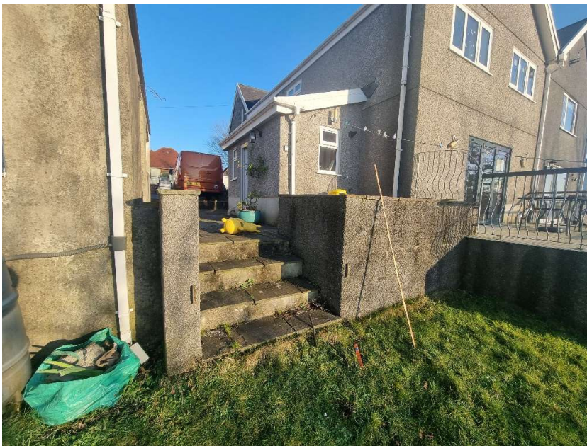
Rear access steps down to lawn with raised patio shown.
