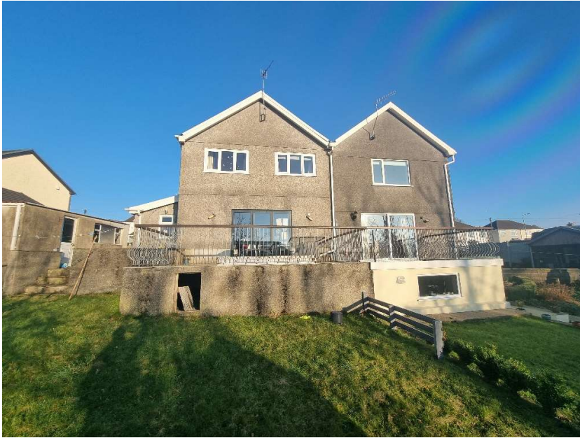
Rear elevation view with lawn, raised patio area and outbuilding shown
