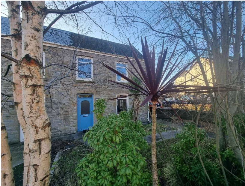
A further view of the front elevation with some mature trees in the foreground.
