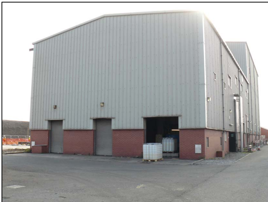
Photograph 11: Existing sludge de-watering building
