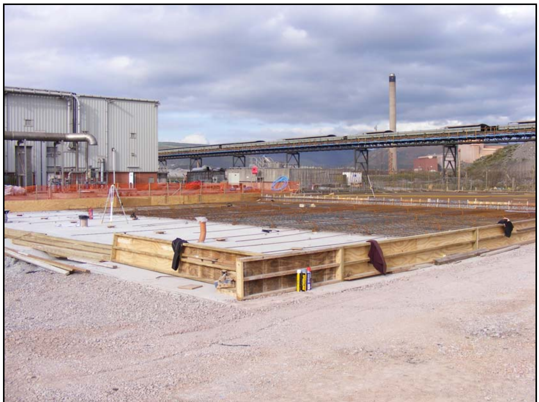
Photograph 6: Concrete slab in preparation for proposed sludge de-watering and storage building, looking north
