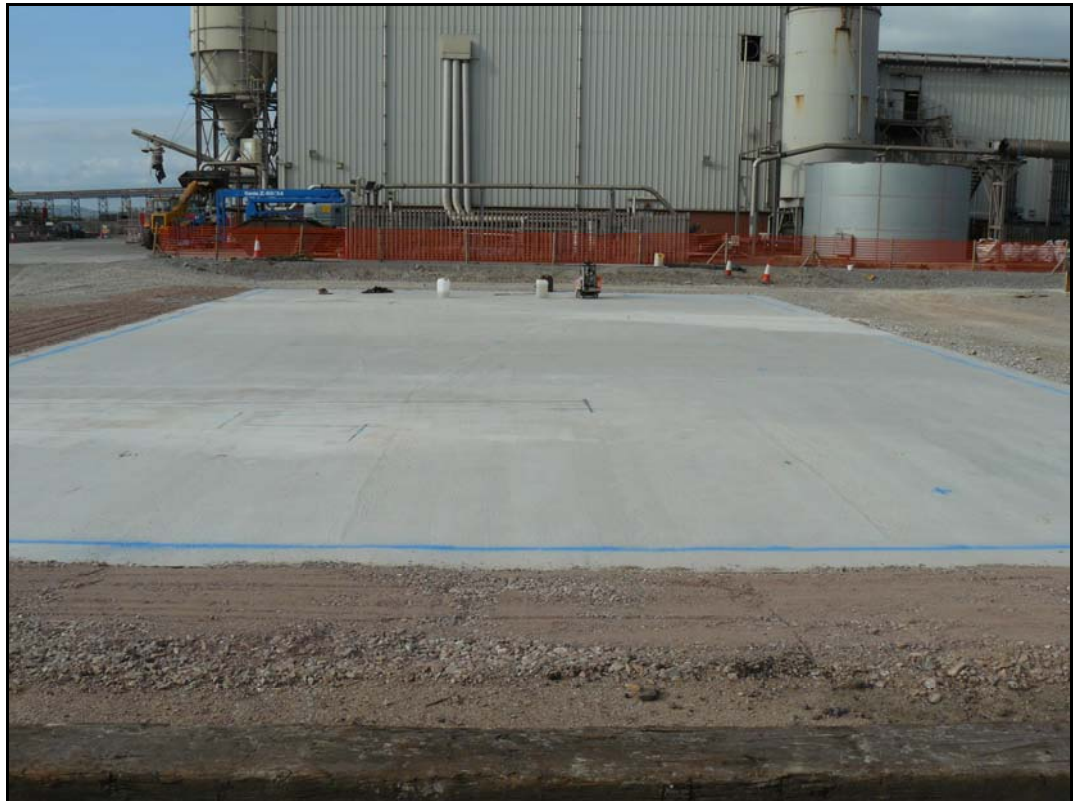
Photograph 5: Concrete slab in preparation for proposed hydrolysis plant and digested sludge storage tank, looking North West
