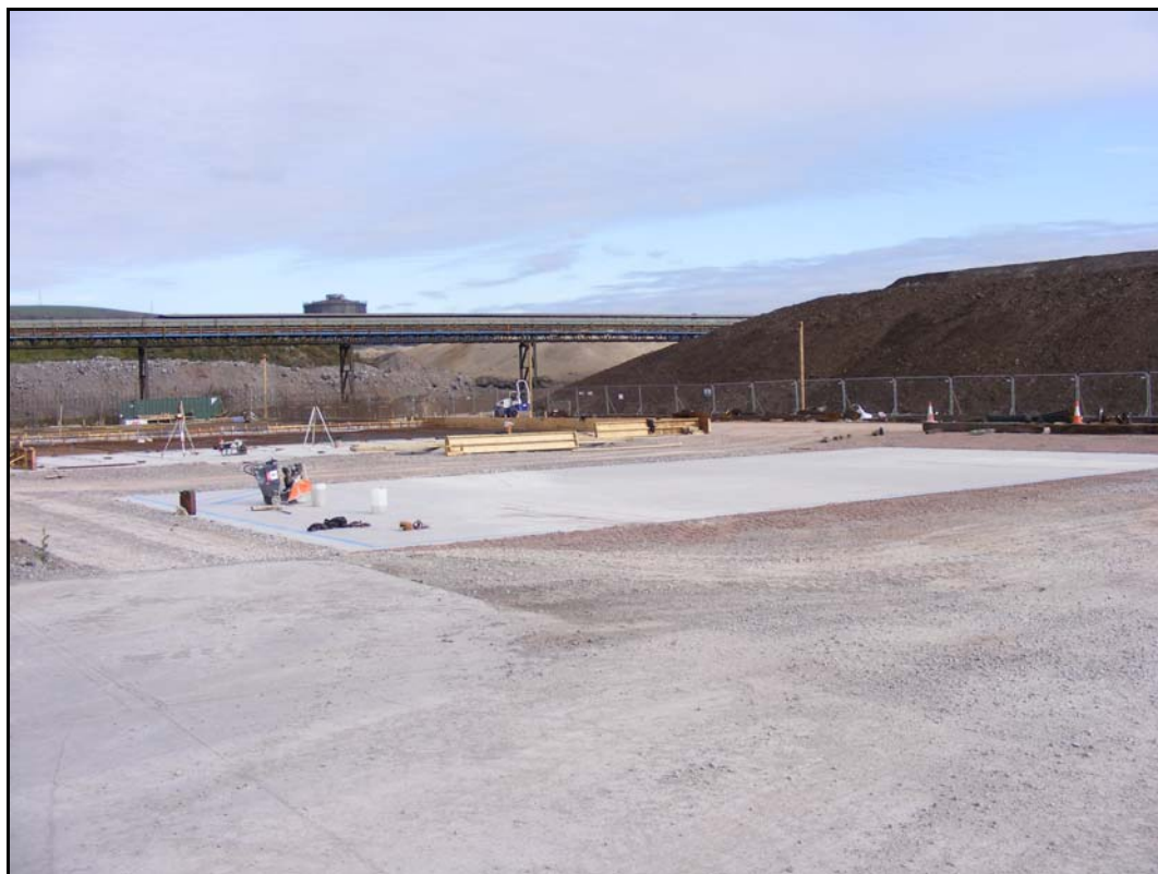
Photograph 3: Concrete slab in preparation for proposed hydrolysis plant and digested sludge storage tank, looking east
