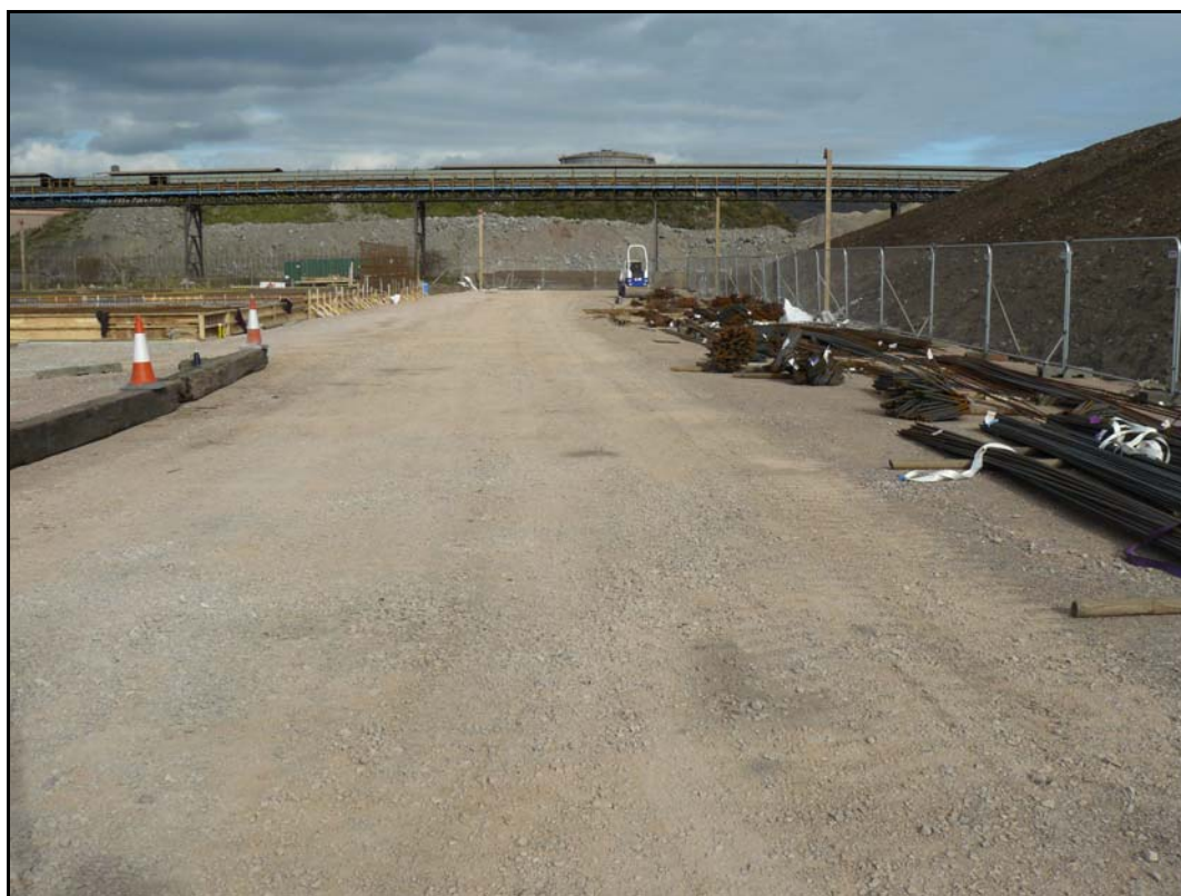
Photograph 4: Proposed access road looking north east
