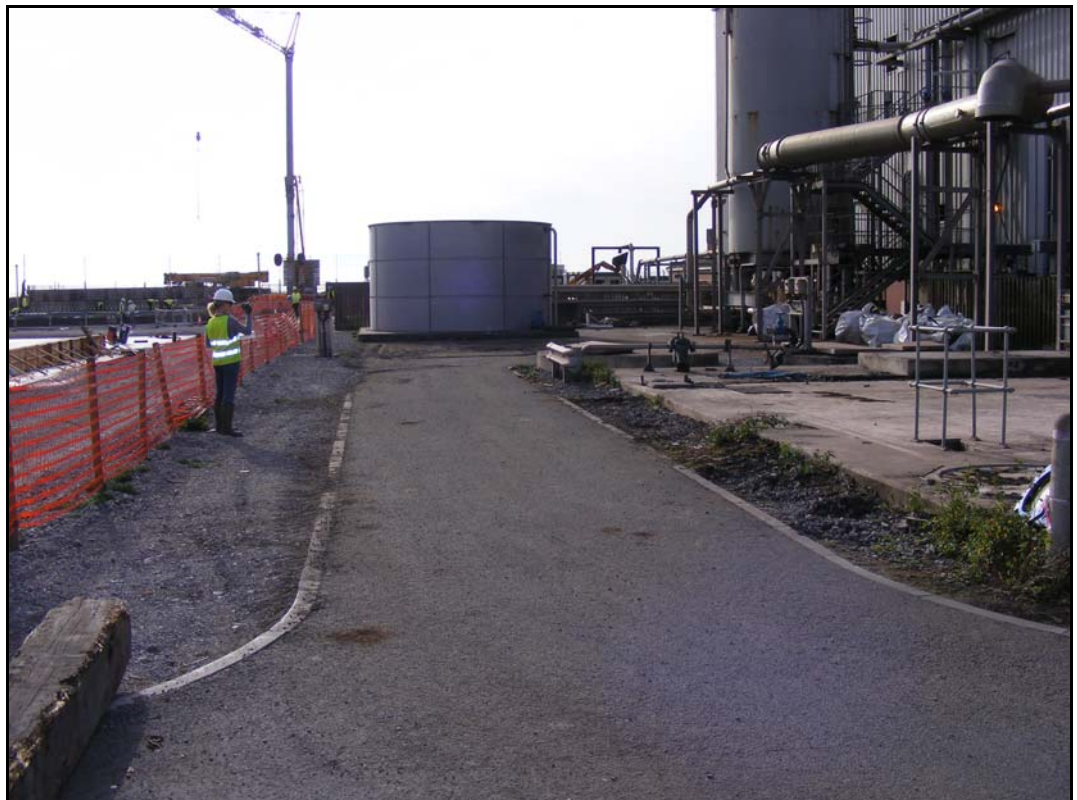
Photograph 8: New access road and relocated liquor balancing tank, looking south west
