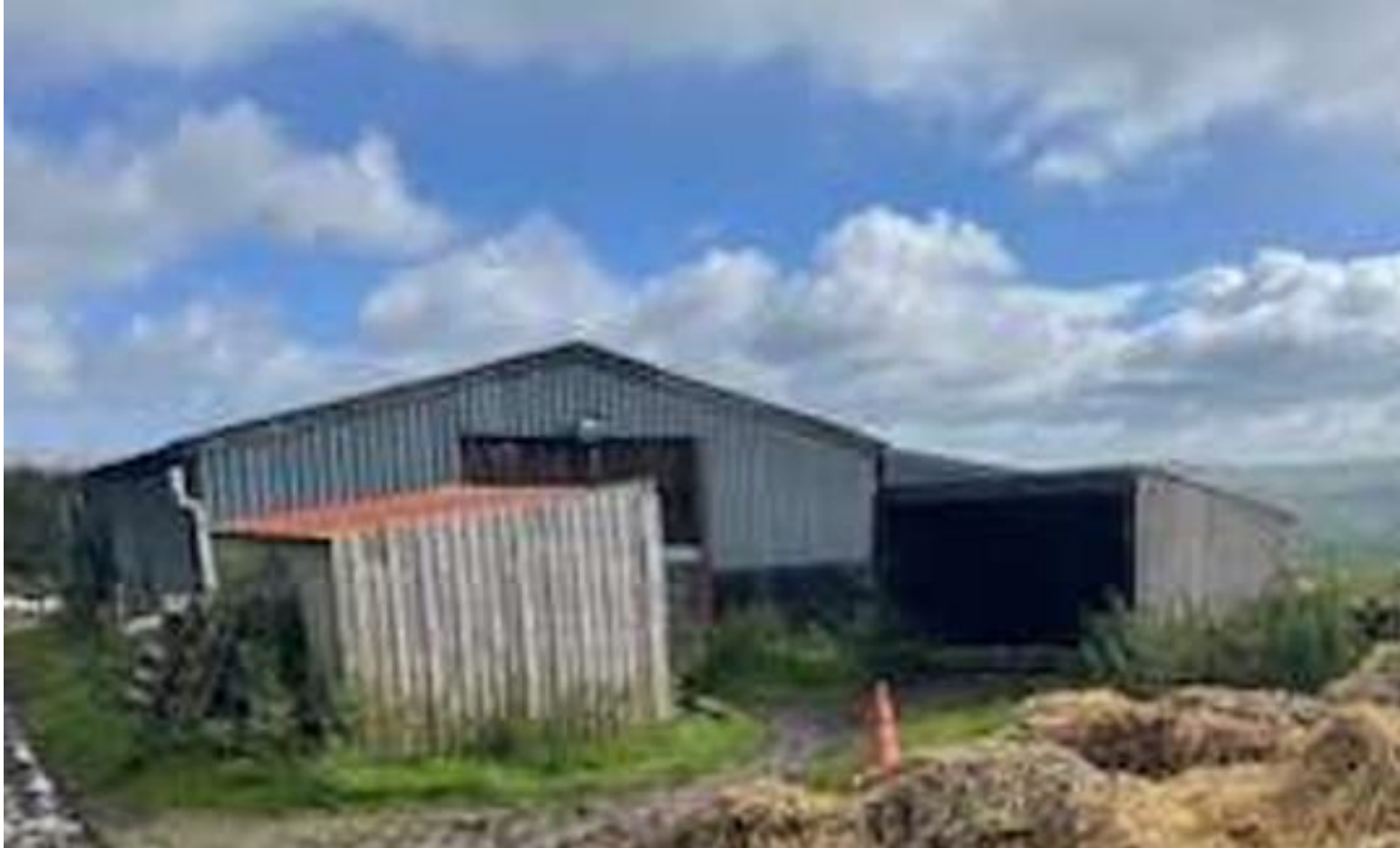
Deri Isaf Farm Storage Shed – Back of barn where planned extension will be (two lean-to storage areas already removed)
