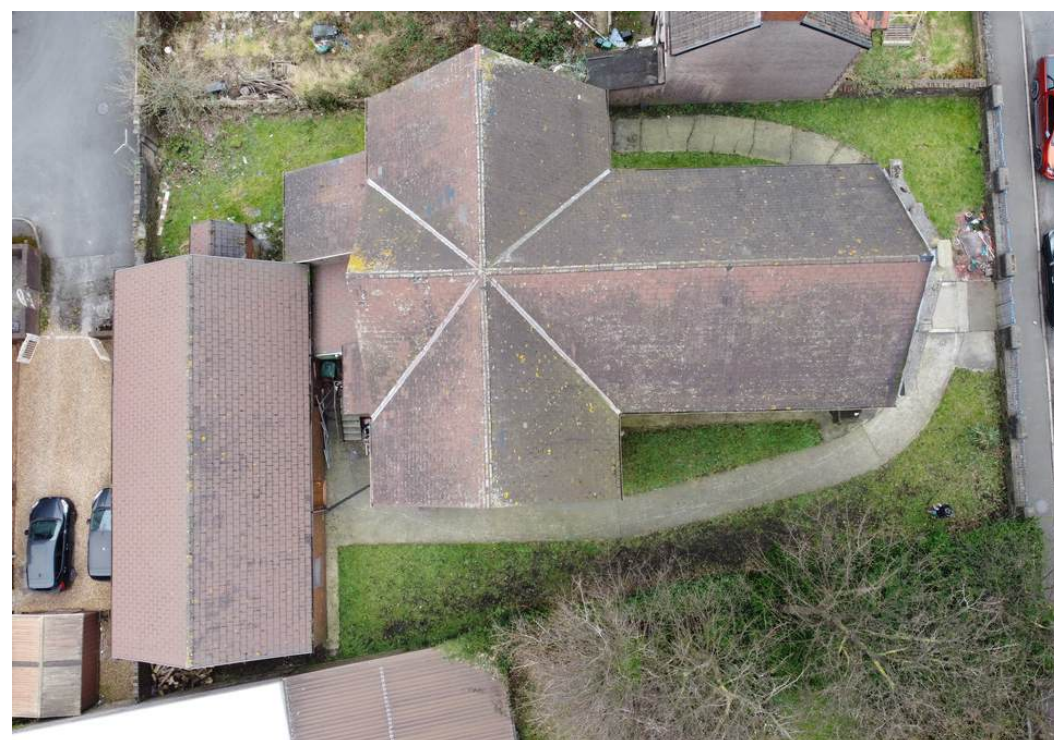
Figure 31 – Church roof and land
