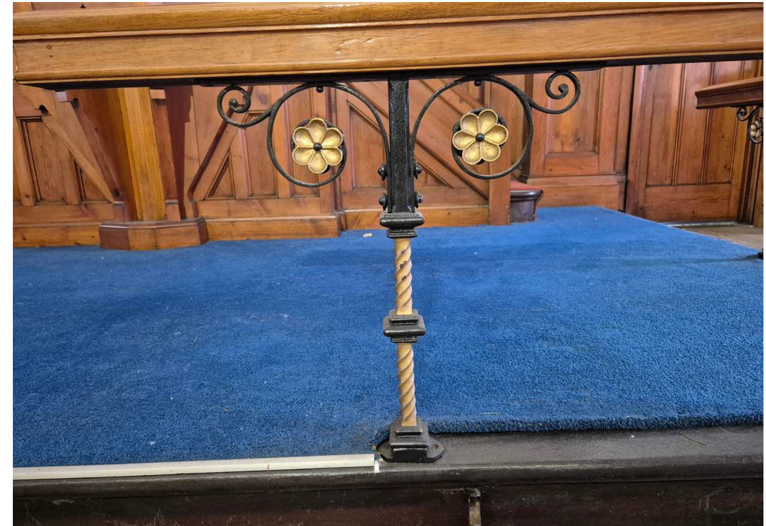
Figure 19 – Decorative steel work to pulpit handrail
