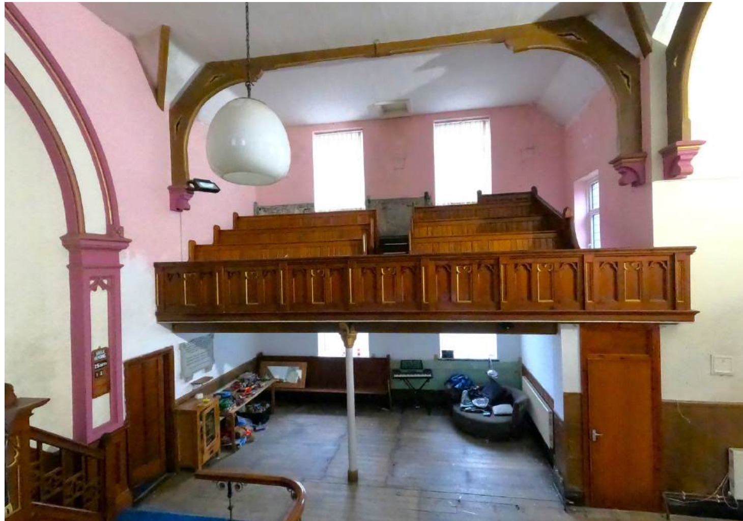
Figure 20 – Balcony with pews and supporting cast iron column
