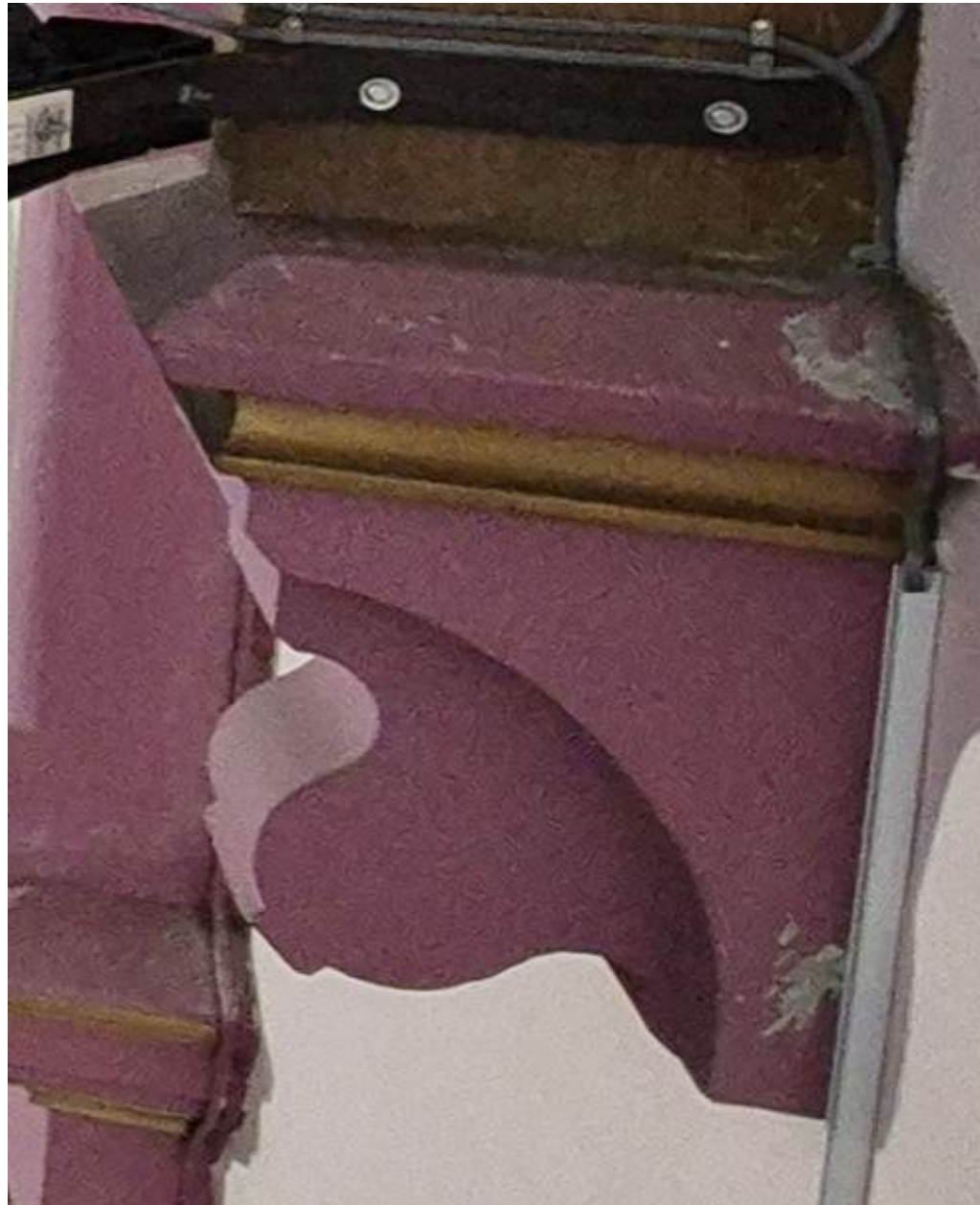
Figure 5 – Decorative corbel stones under all trusses
