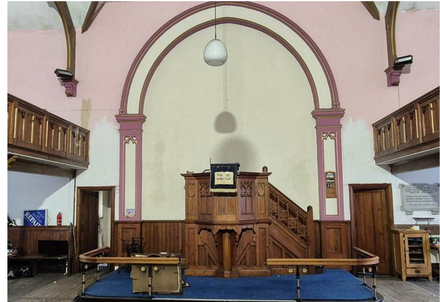
Figure 23 – Running mould lime plaster work
