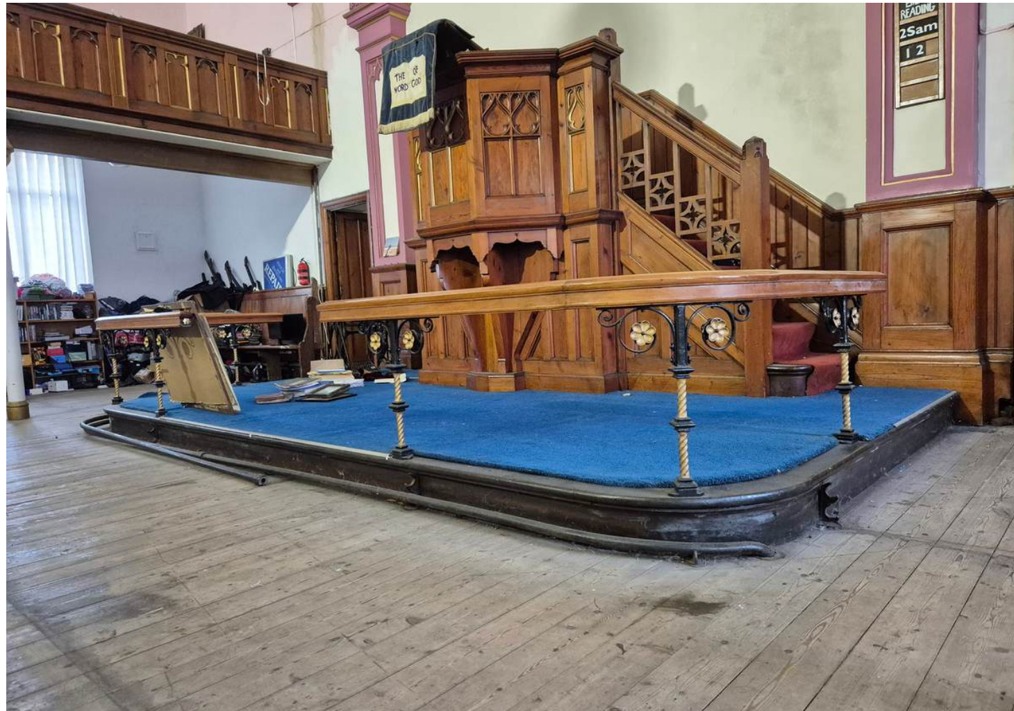
Figure 18 – Pulpit, raised platform and handrail
