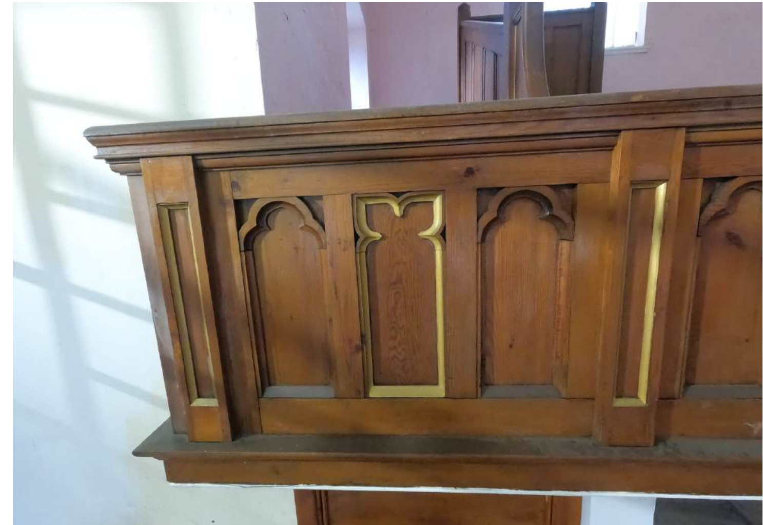
Figure 21 – Decorative panelling to the balcony's
