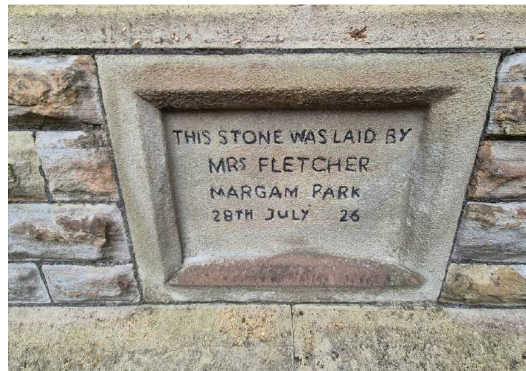
Figure 12 – Plaque right of front door
