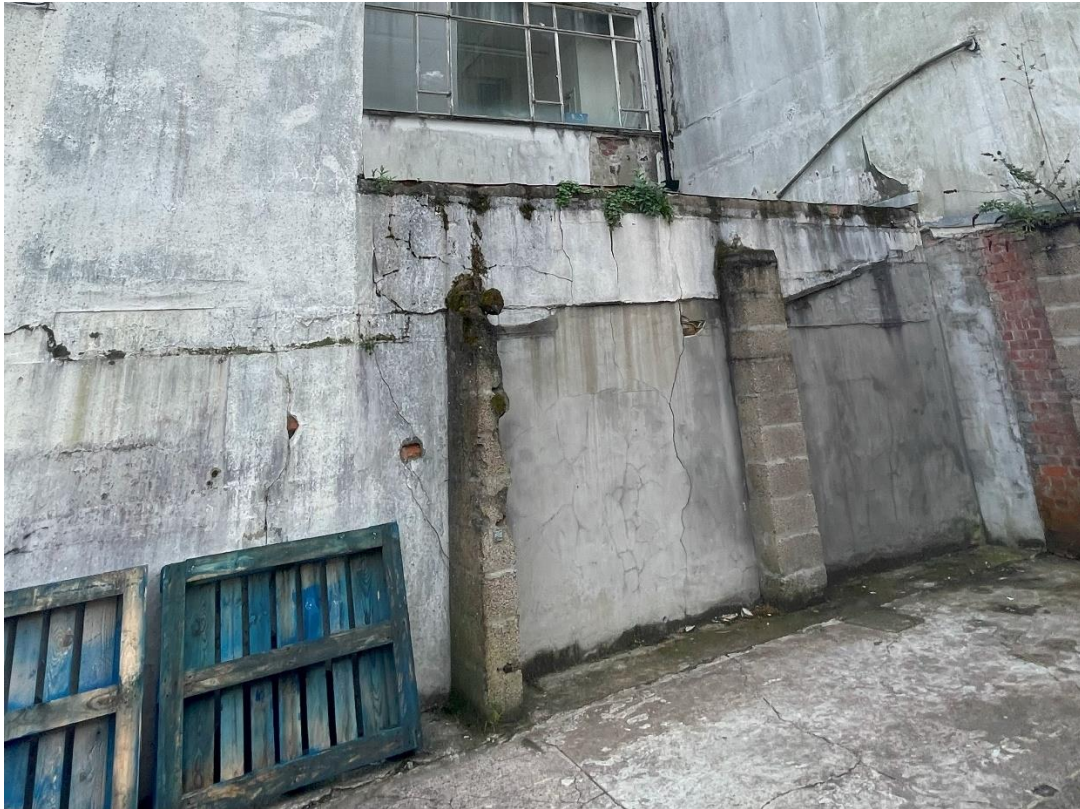
Photograph 9 –Lower rear section to be removed
