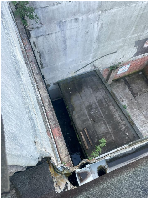
Photograph 6 –Freestanding lower rear section
