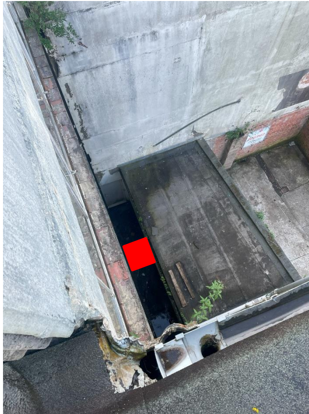
Photograph 11 –Location of manhole at rear
