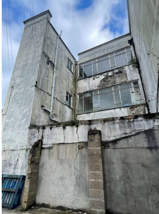
Photograph 1 – Rear of Peacocks Neath
