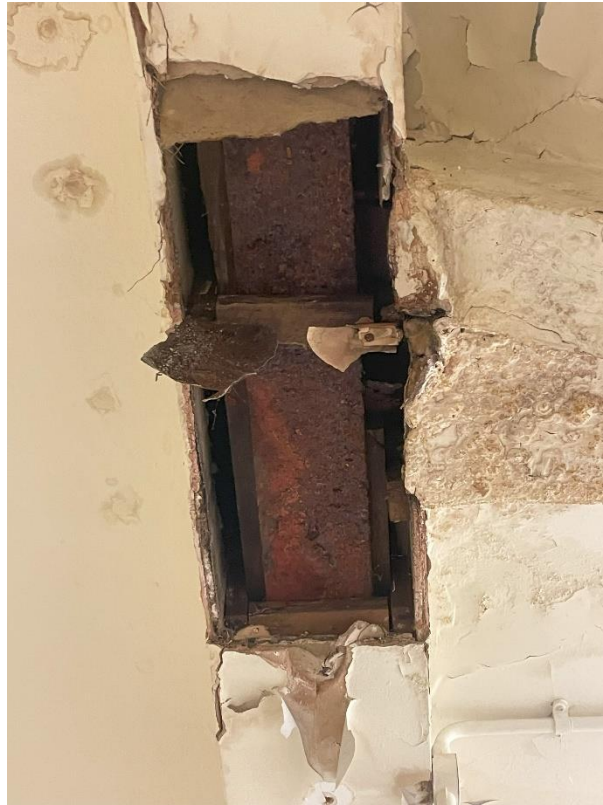
Photograph 7 –Exposed section of steelwork beam spanning laterally
