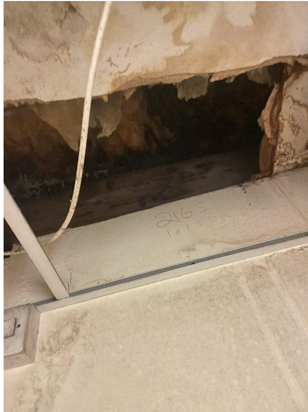
Photograph 3 – Formation of flat roof
