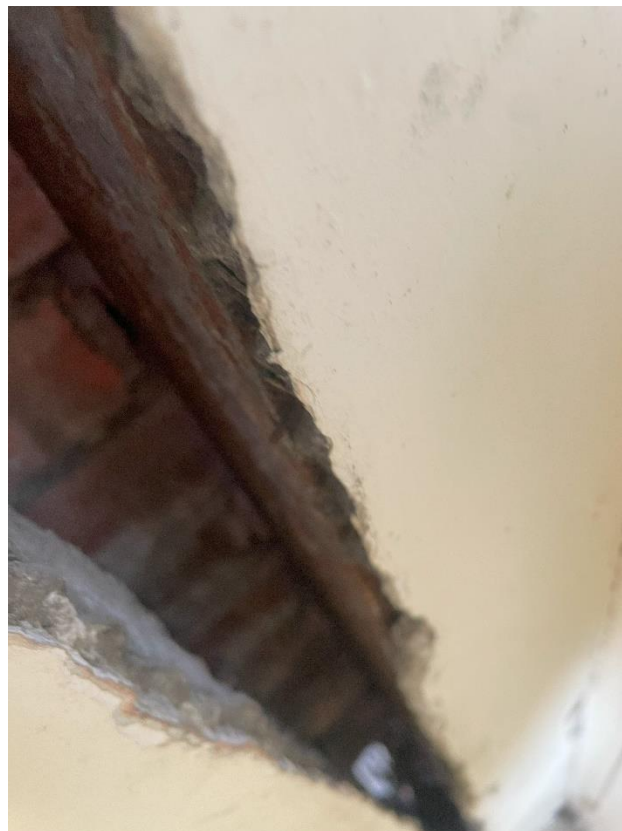
Photograph 4 –Column encapsulated in wall between proposed demolished area and retained area
