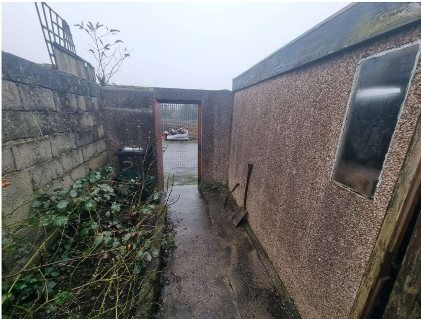
View of rear area including rear access gate, existing garage and existing blockwork boundary wall to left side neighbour
