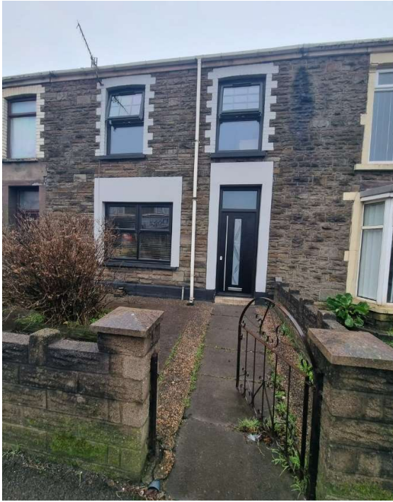
View of front elevation including front yard area
