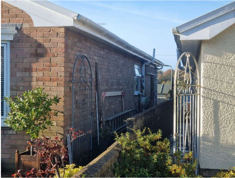
View of boundary to right hand side neighbour with low blockwork wall. This will remain unaltered.
