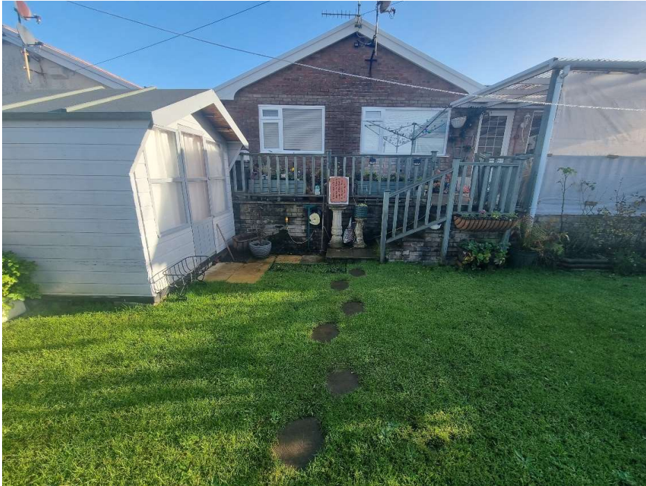
Rear garden view including lawned area, existing raised patio and existing lean to covered area
