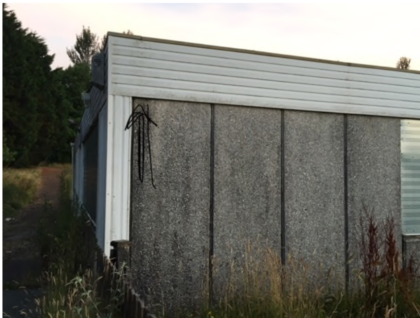
Southern elevation, bat re-entry
