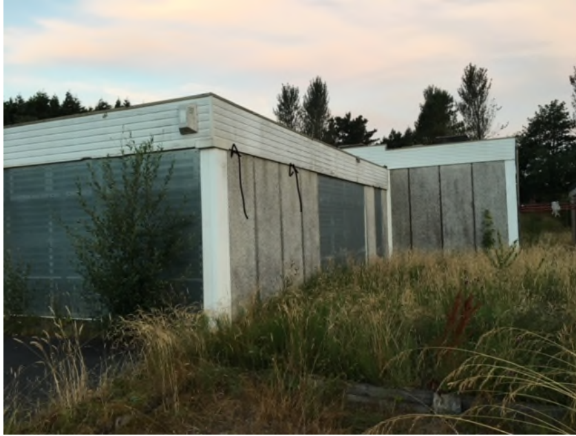
South eastern elevation bat re-entry
