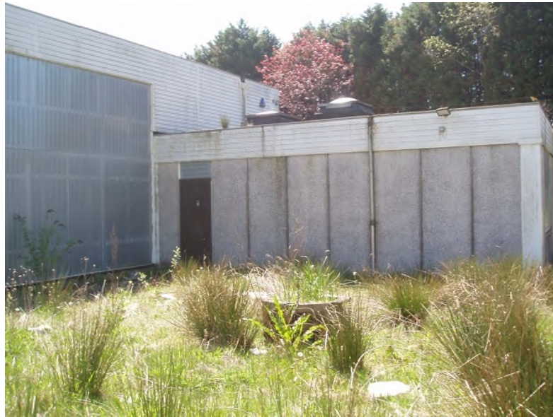
School front and main entrance (sealed)
