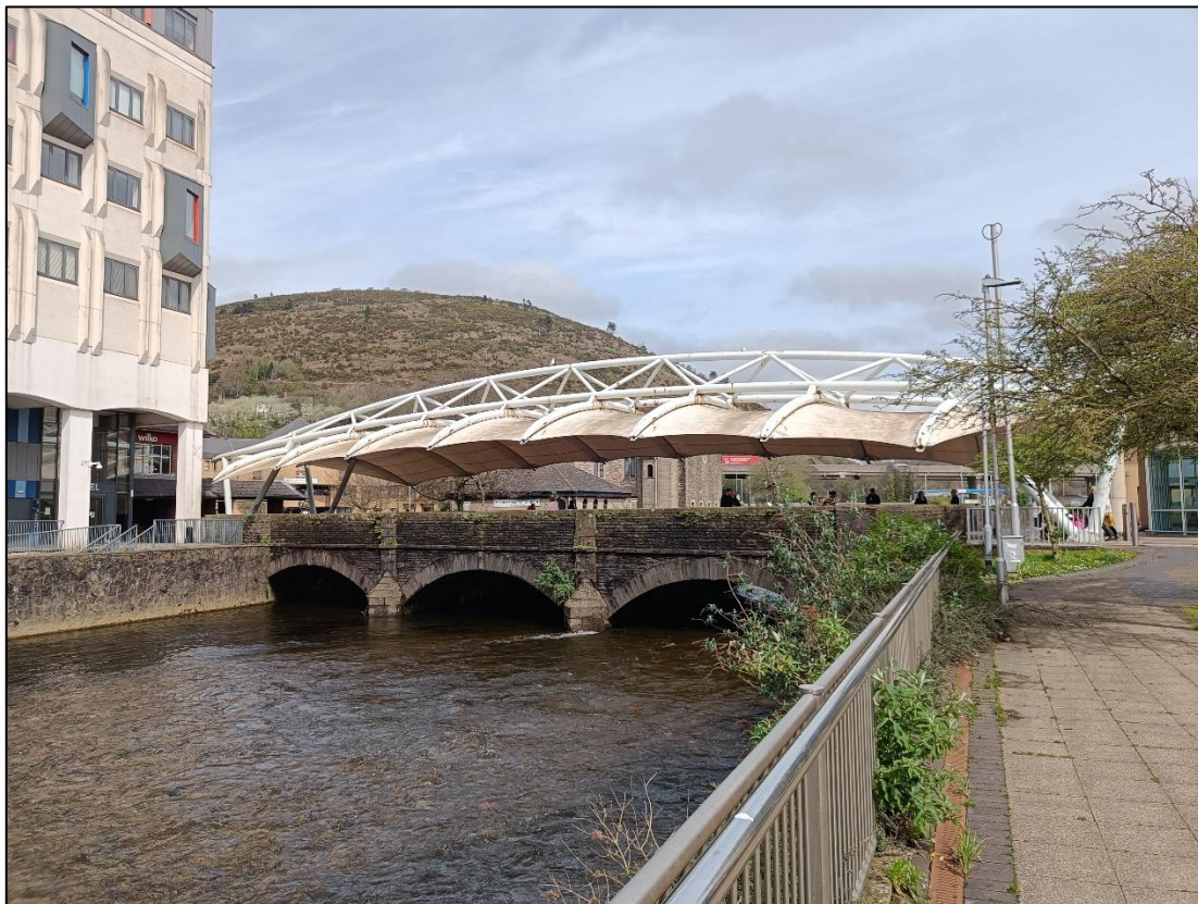
Figure 9. View north of the listed bridge. The chapel is visible beyond the bridge.
