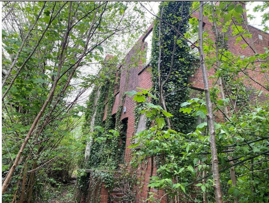
Plate 3: Southern and eastern elevation of main house
