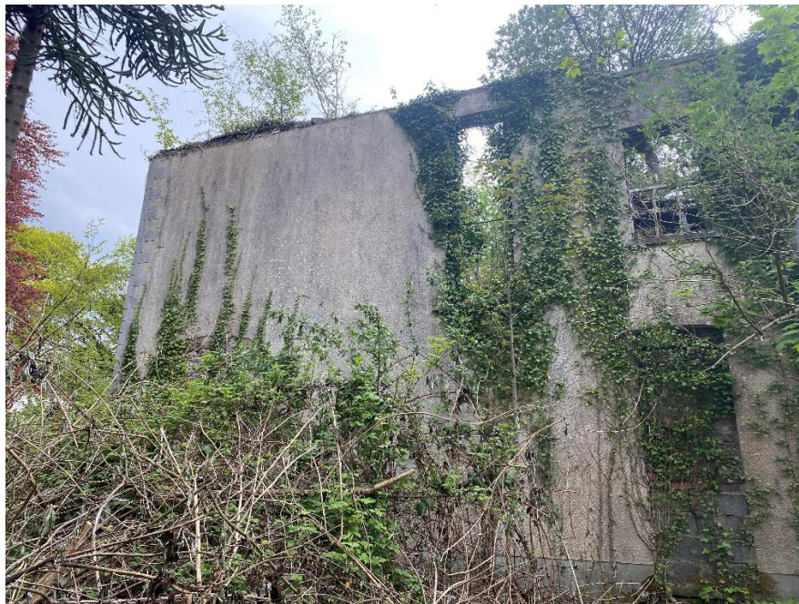
Plate 2: Western elevation of main house
