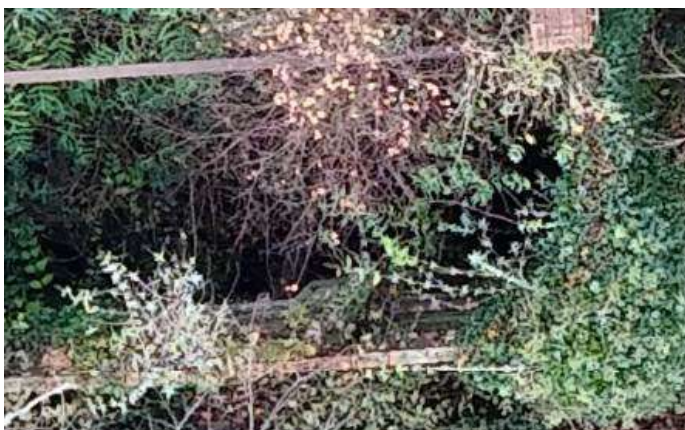
Drone footage showing slenderness at the head of the north, brick wall and steel beams in place
