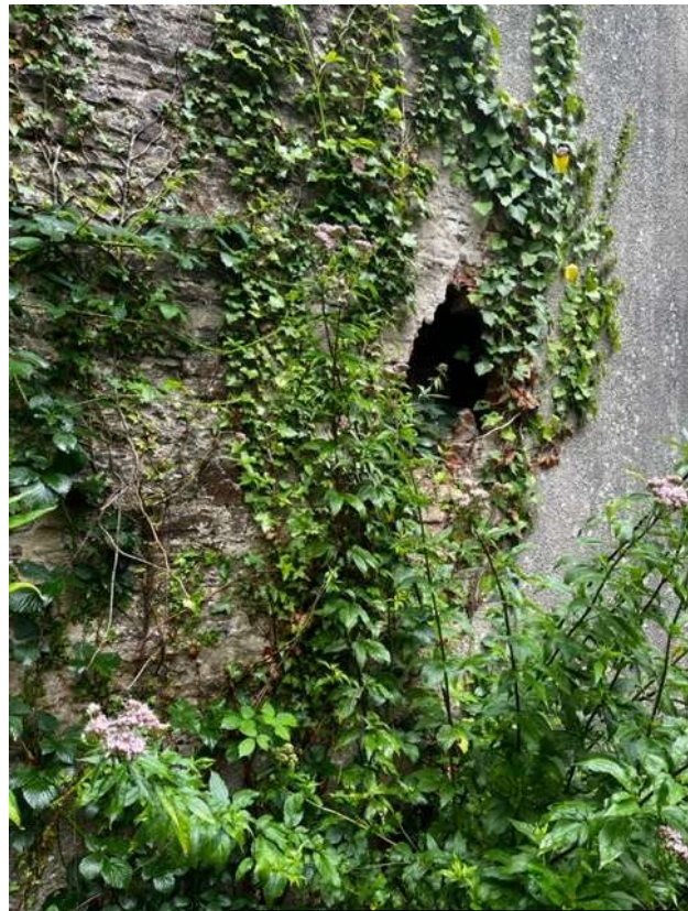
West elevation - July 2023
