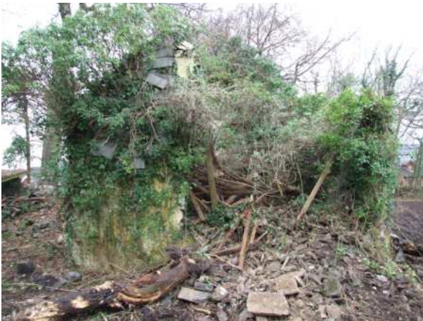
20. The outbuilding immediately to the rear of house; west gable c.2014
