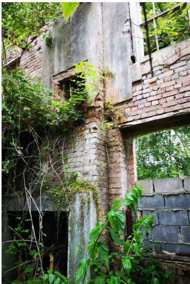
13. The interior of the brick extension; Sept 2019
