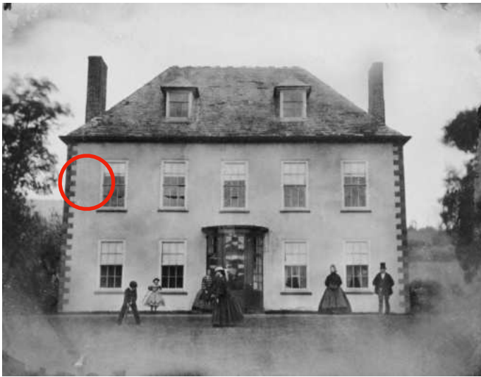
1. Tyn yr Heol House c.1890s; original front elevation, stone roof, semicircular central timber porch and stacks
