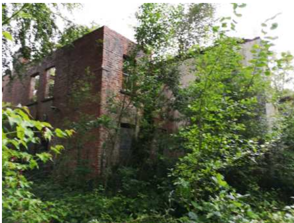
9. The brick extension; Sept 2019
