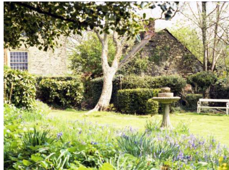
16. View of the west gable of outbuilding to the rear of the house c.1980
