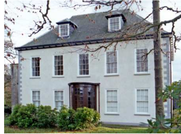
4. Tyn yr Heol House c.1980s; extension to side, cement render, lost stacks and replacement slate roof
