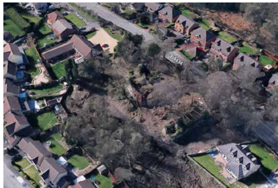
Photo 5 Aerial view looking west
