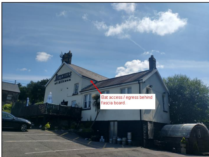
Photograph 1. Main building south elevation.
