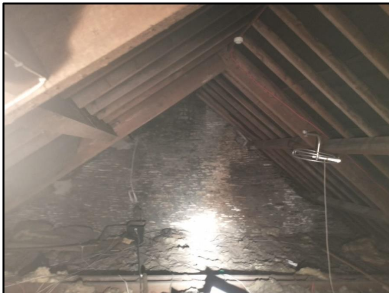
Photograph 7. Main building attic space south side.
