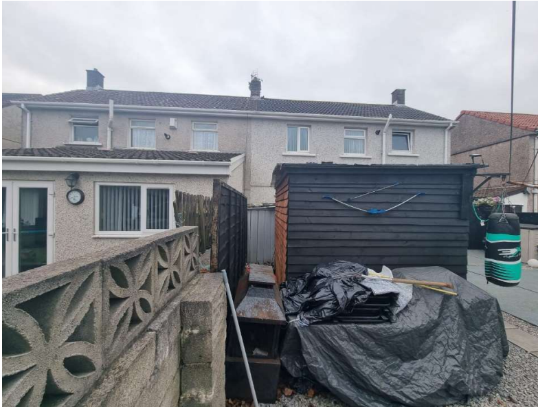
Rear elevation view showing timber and blockwork boundary wall and existing outbuilding.
