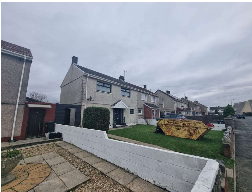
Front elevation and side view showing blockwork boundary wall and front garden area
