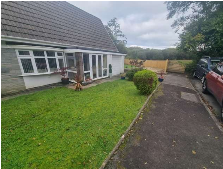
Front area view from road
