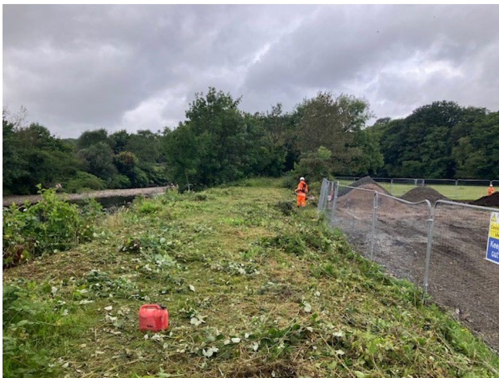
Figure 2 – Vegetation clearance undertaken along the Flood Bund in February 2024.
