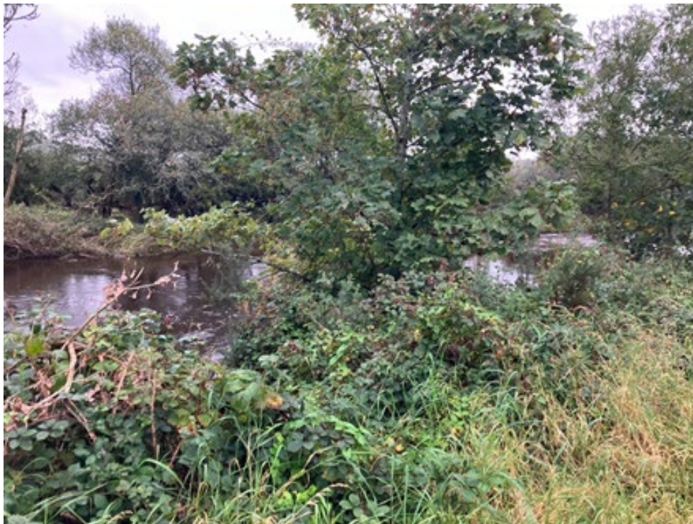
Figure 1 - Outfall Headwall location September 2023.
