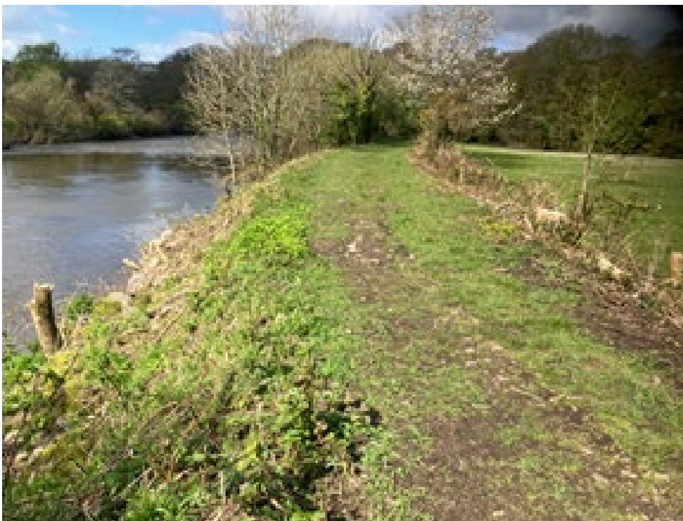
Figure 3 - Outfall Headwall location in April'24 following the clearance works in February 2024
