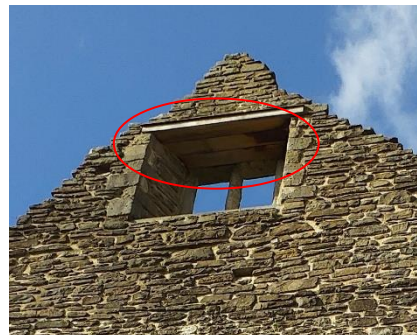
Wooden lintel with potential for roosting/hibernating bats
