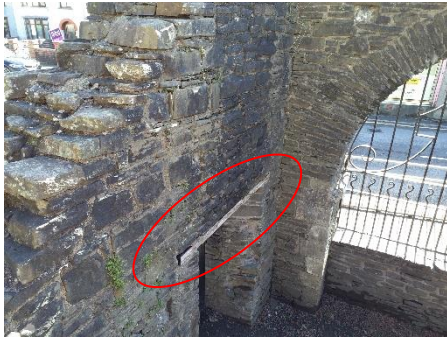
Wooden lintel with potential for roosting/hibernating bats (Gatehouse)
