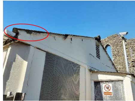
Modern building with gaps to the verge with potential for roosting bats
