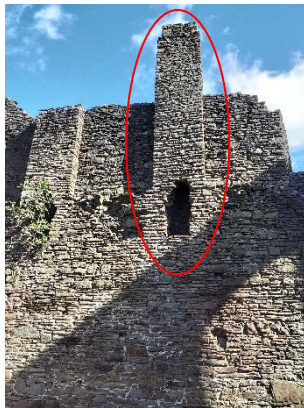
Chimney with potential for roosting bats
