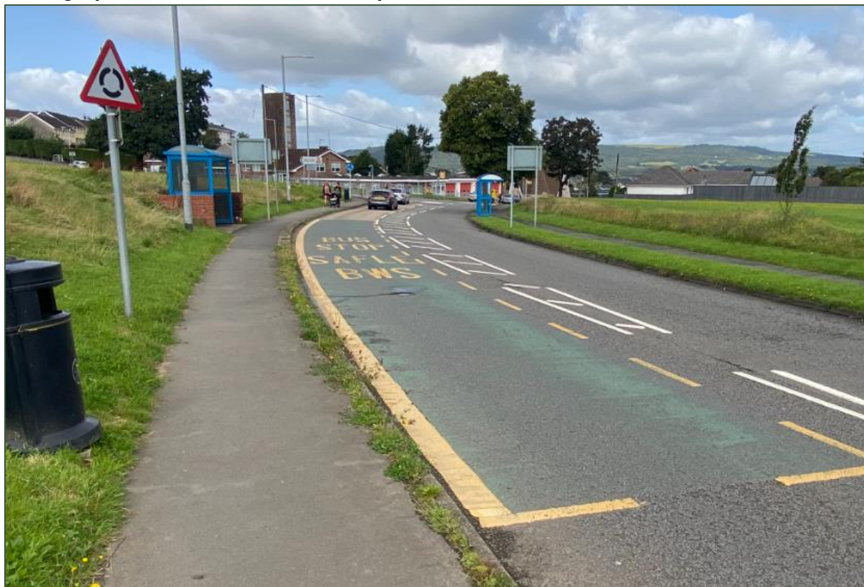
Photograph 2.4 – Fire Station Bus Stops
