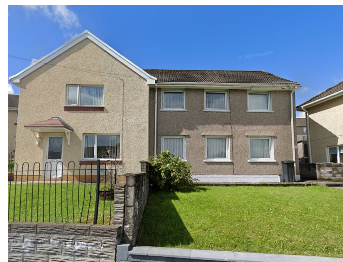
Dwellings located at Valley View.
