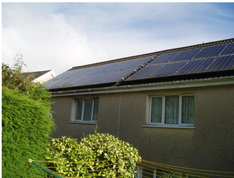
The rear western elevation.
