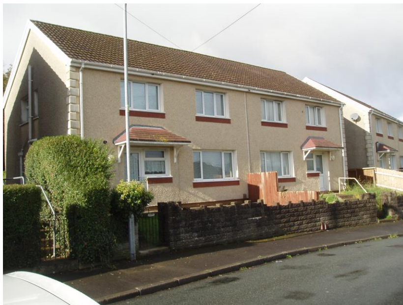
The front, eastern elevation.
