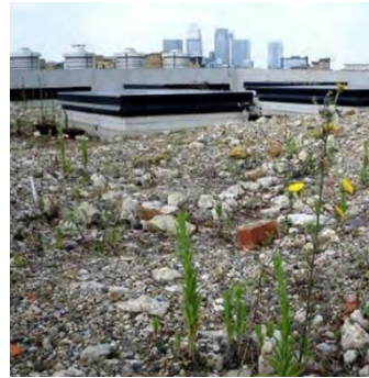
Self-seeded gravel-based rain garden
