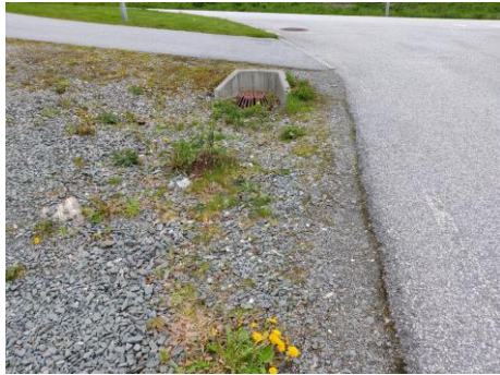
Roadside filter drain with self-seeded vegetation (JBA Consulting)
