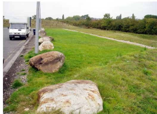
Filter strip providing treatment to road runoff prior to surface water entering filter drain (Susdrain image)
