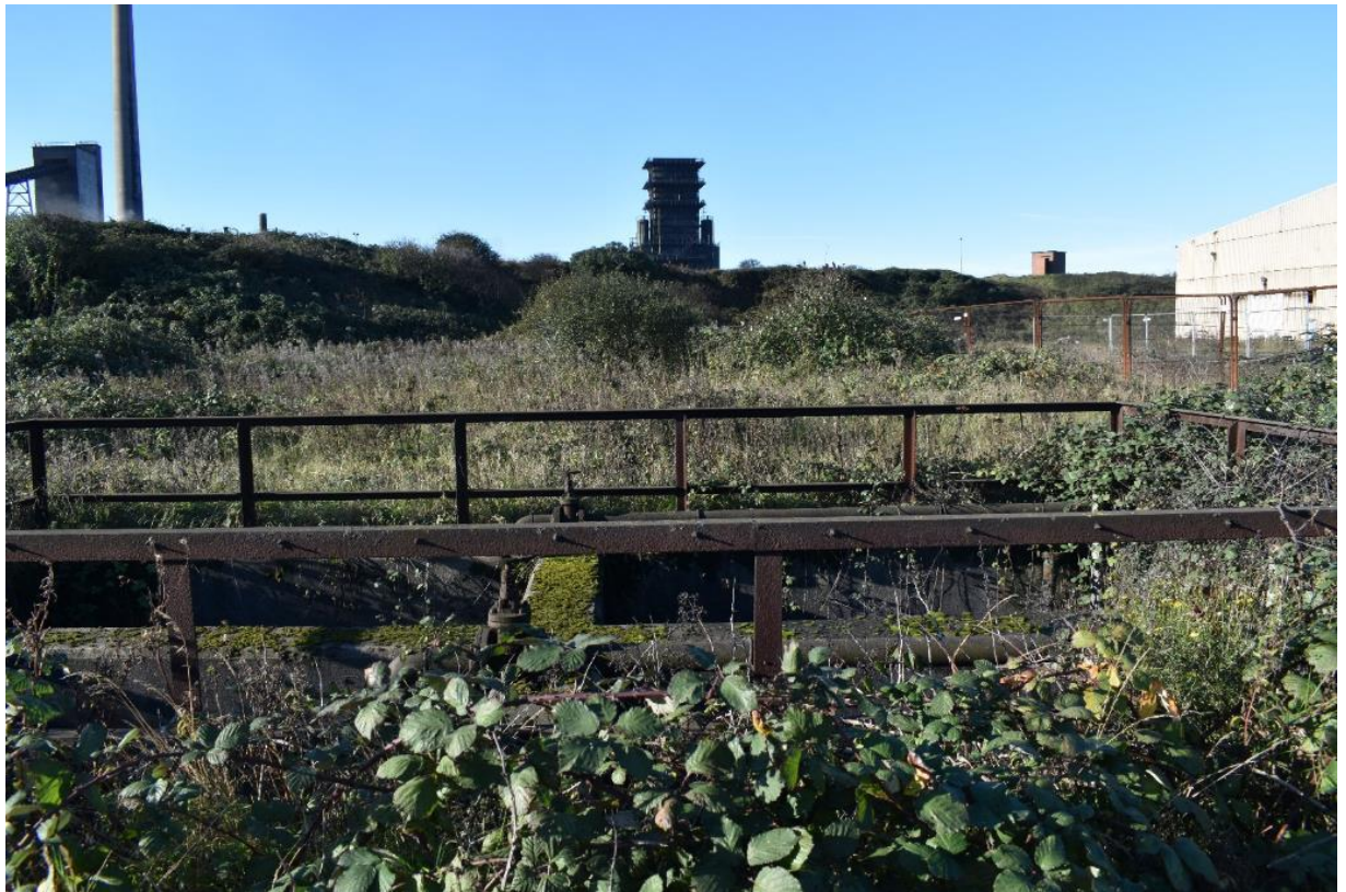
Illus 10. Disused concrete lined pit, facing west
