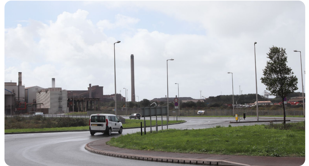
Figure 48: Site access road at Harbour Way roundabout
