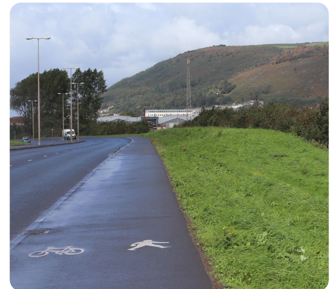
Figure 50: Shared foot/cycle way on Harbour Way
