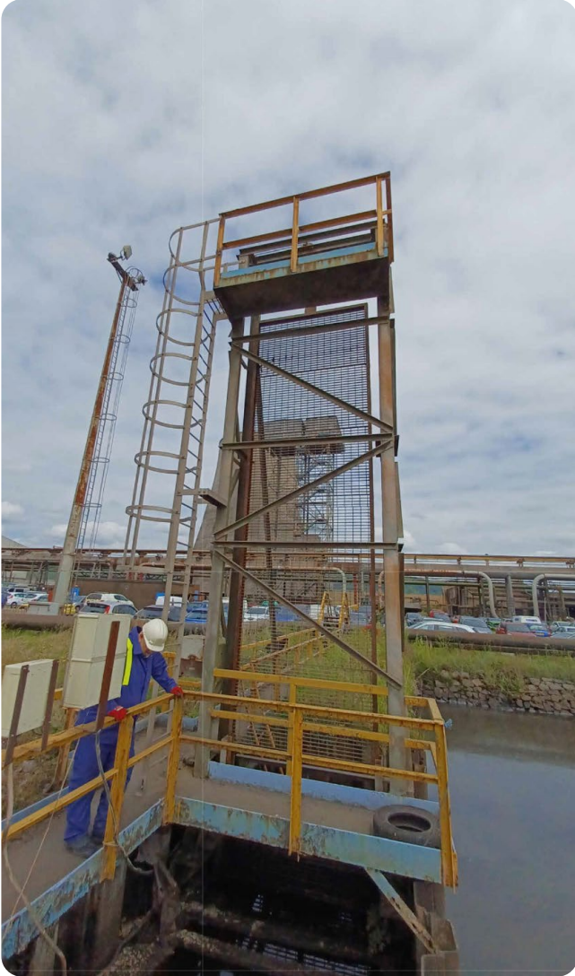
Figure 79: 1O Inlet Structure
