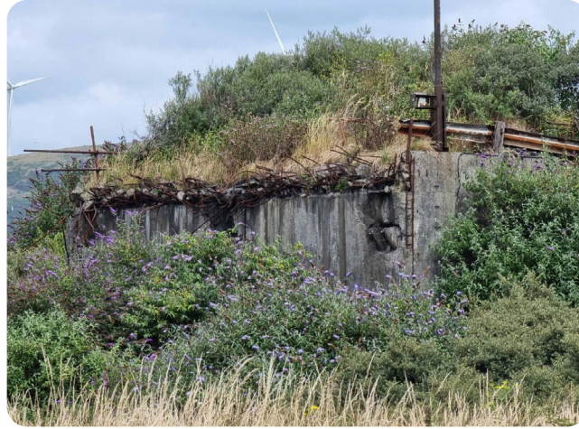
Figure 80: 1Q Concrete Abutments
