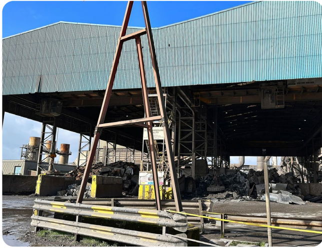
Figure 65: 1A Scrap Storage Shed
