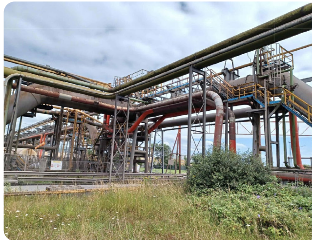
Figure 77: 1P BF Gas Pipe Rack (Partially Removed)
