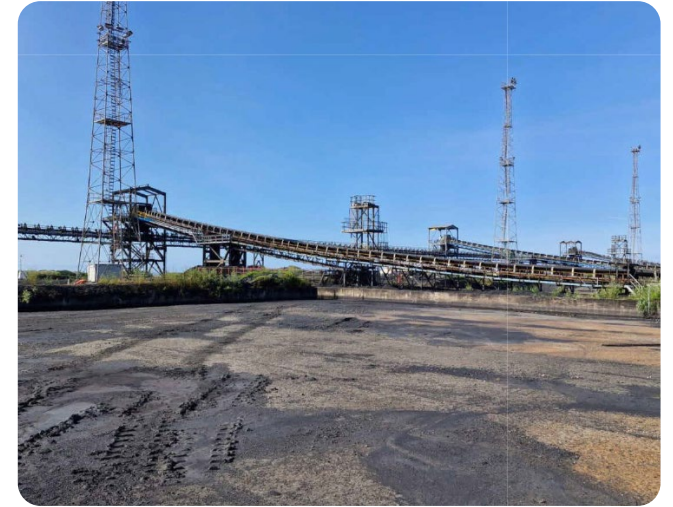
Figure 76: 1N Coal Conveyor Superstructure
