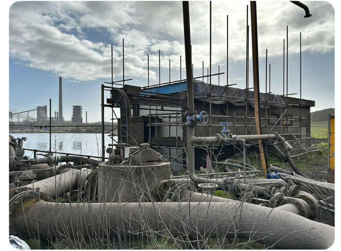
Figure 66: 1B Existing Pump House
