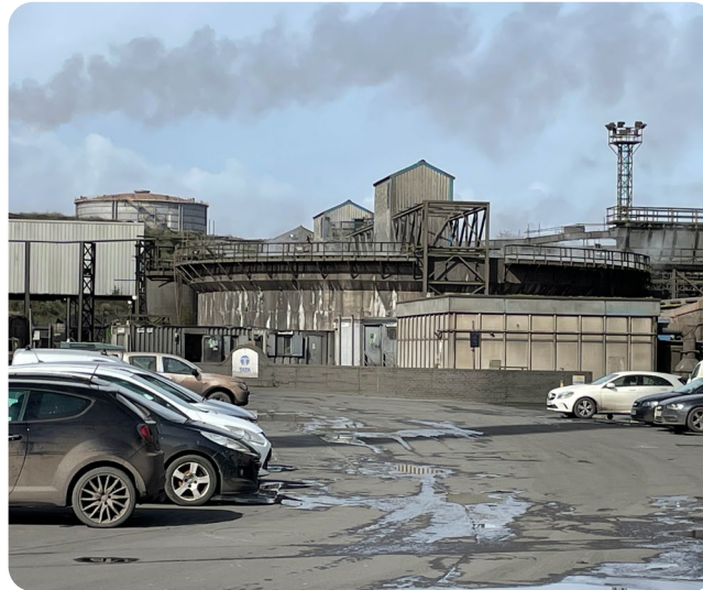
Figure 33: Parking adjacent to the BOS plant
