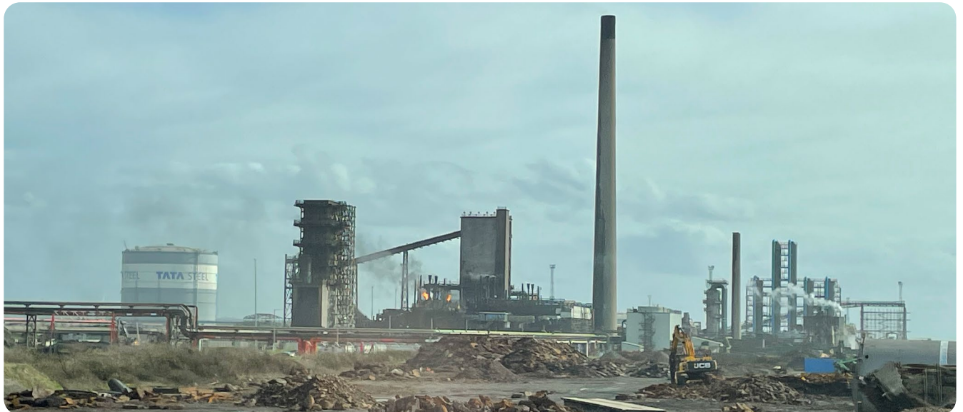
Figure 35: Coke ovens (now decommissioned)
