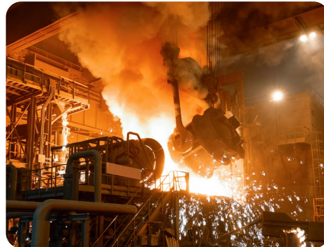
Figure 17: Ladle metallurgy furnace (Getty Images)
