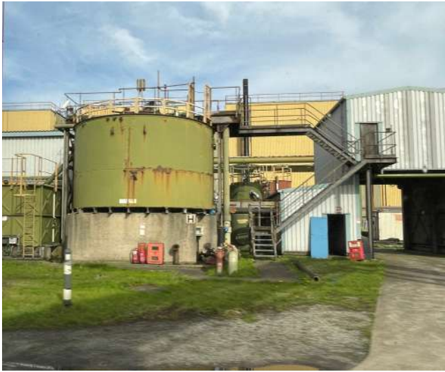
Figure 7: Rolling Mill Exterior
