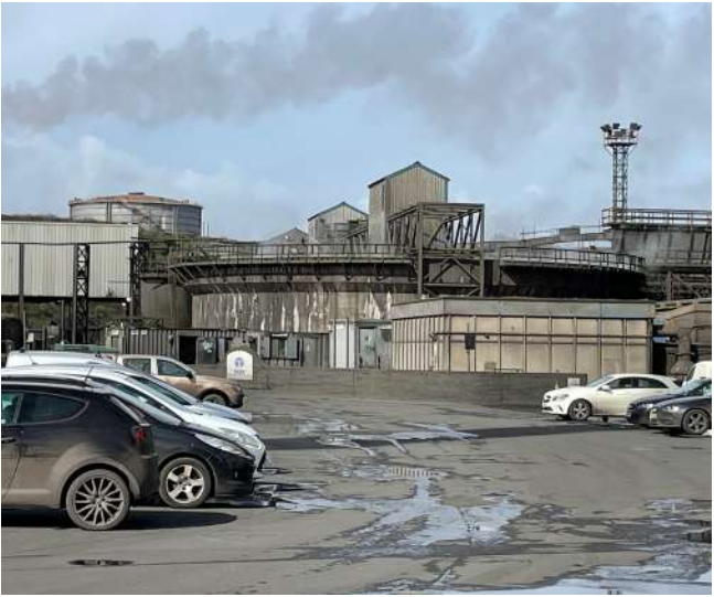
Figure 9: Parking adjacent to the BOS Plant
