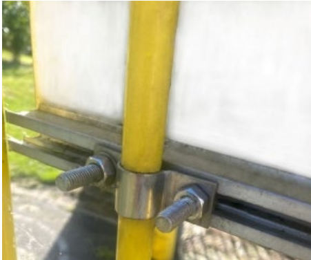
Photograph 4 – Back view of proposed fixing method
