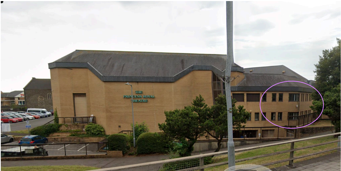
Figure 12: Windows on existing building which could be affected by external plant noise.
