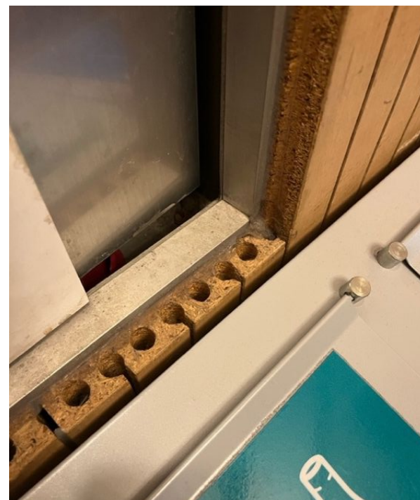
Figure 7: Cut-away view of existing timber wall panels
