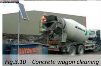
Fig.3.10 – Concrete wagon cleaning
